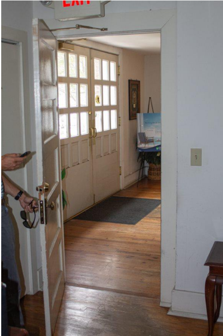
Photo 17 Front entrance detail, taken from the perspective of the northeast, first-story office looking south. Note ca.-1998 double-door, original floorboards, and historic interior door.
