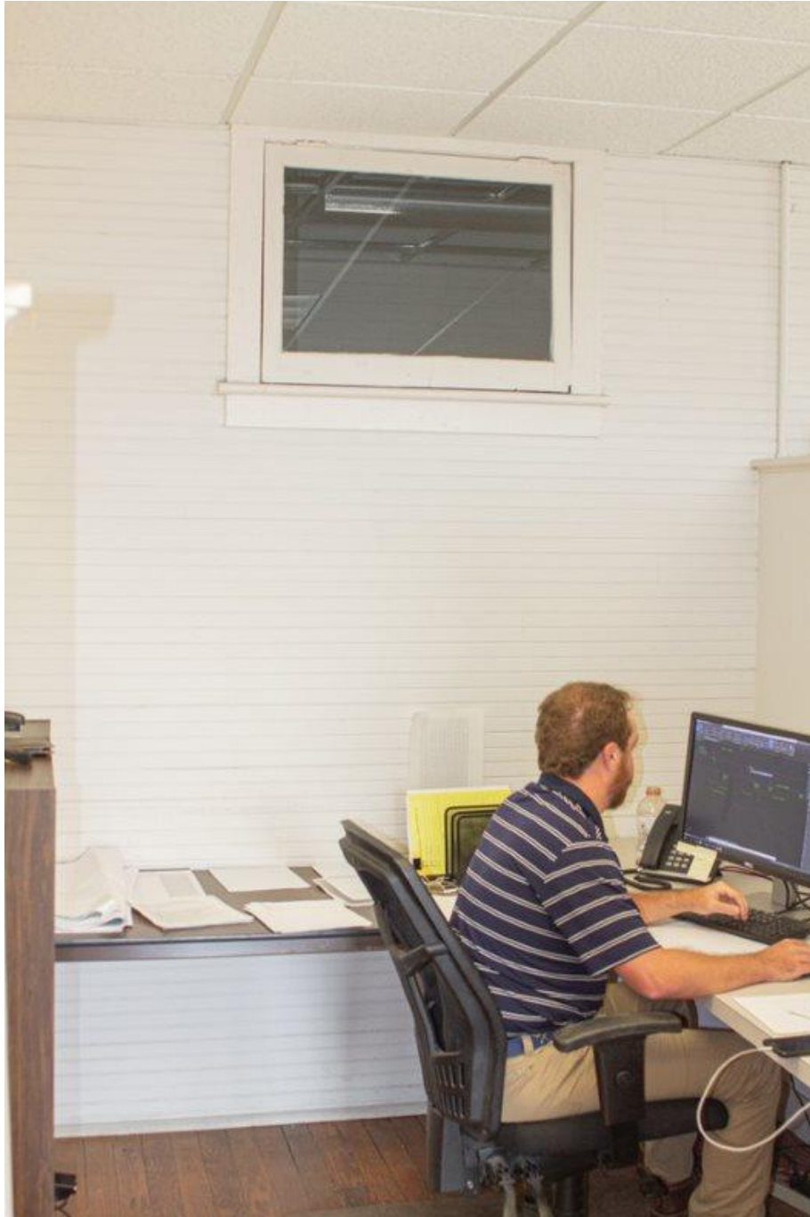
Photo 30 Second-story west office, looking east. Note original beadboard paneled wall and awning-style ventilation window.
