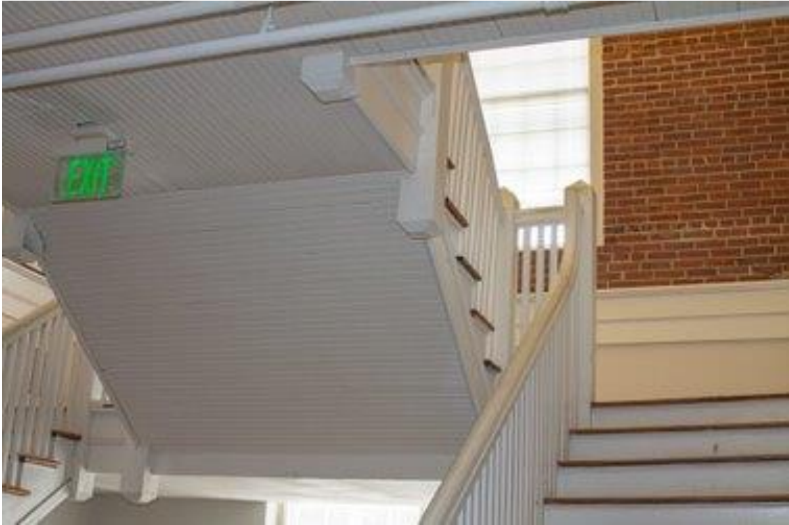
Photo 32 Third-story stair landing. Note exposed brick wall and beadboard on underside of stair stringer.
