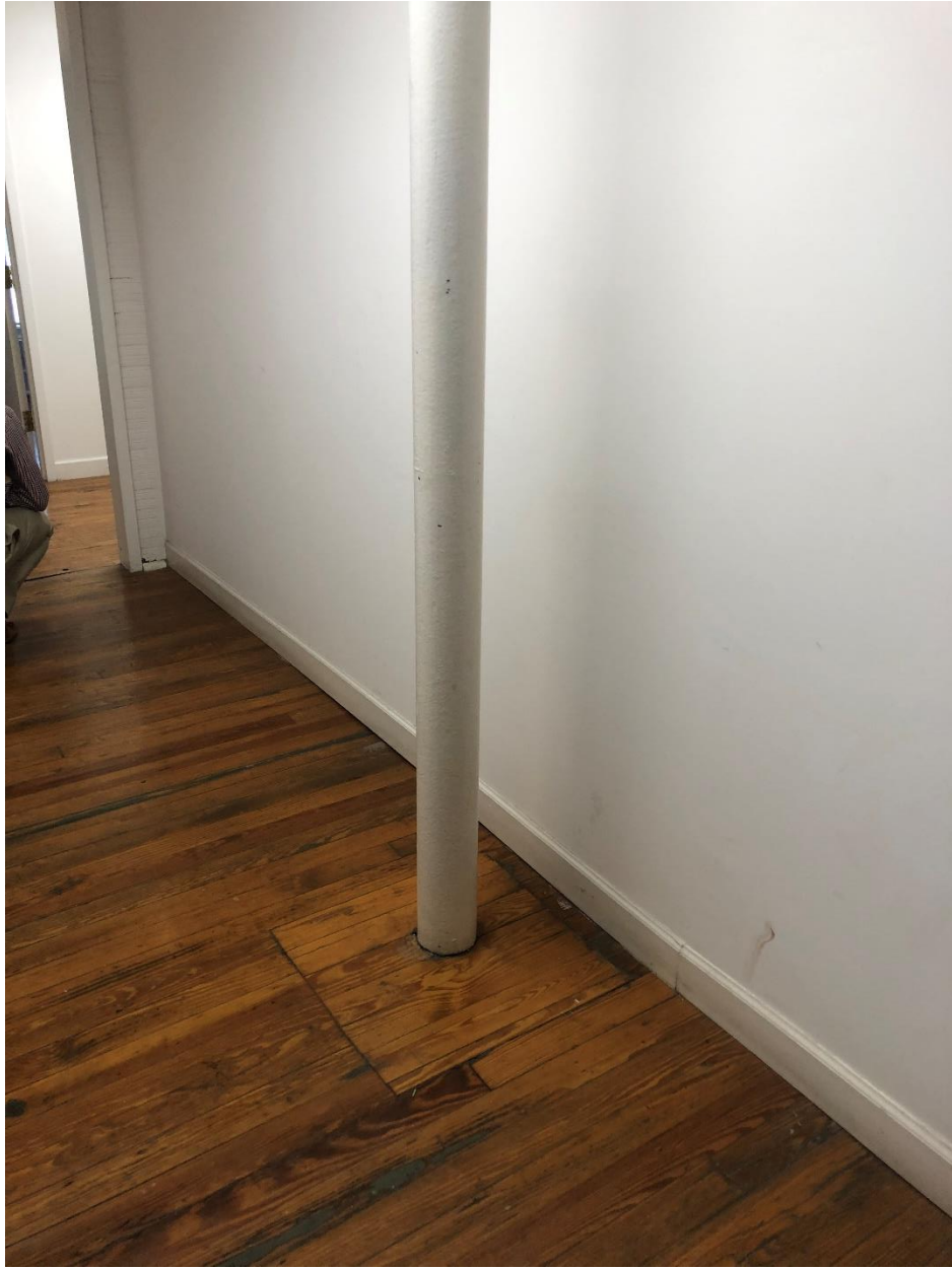
Photo 41 Southwest office detail. Note pipe column of unknown date.
