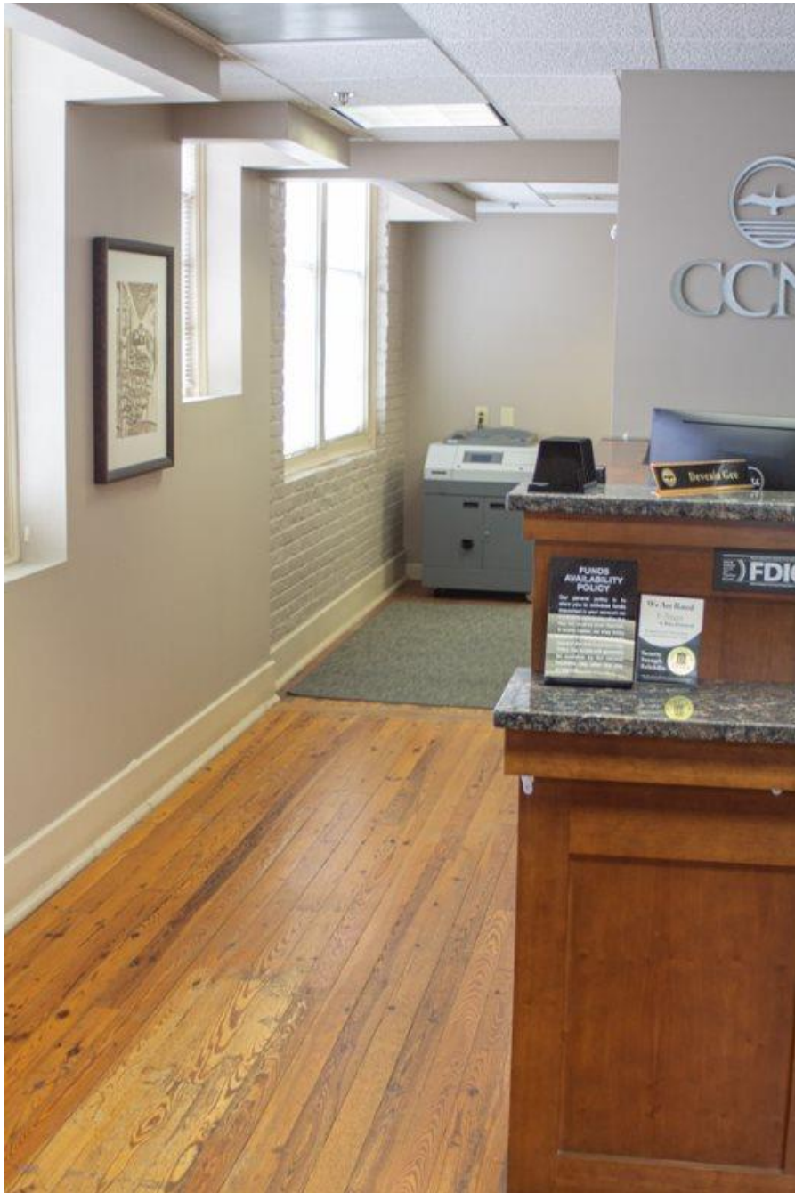
Photo 21 Southeast office detail, taken from the perspective of the southeast, first-story office looking west. Note transition from sheetrock walls to exposed, painted masonry wall.
