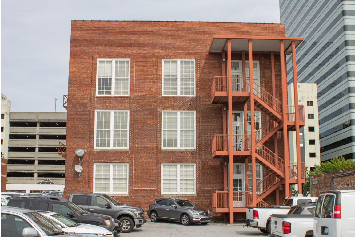
Photo 6 – West elevation illustrating three-story structural steel staircase.
