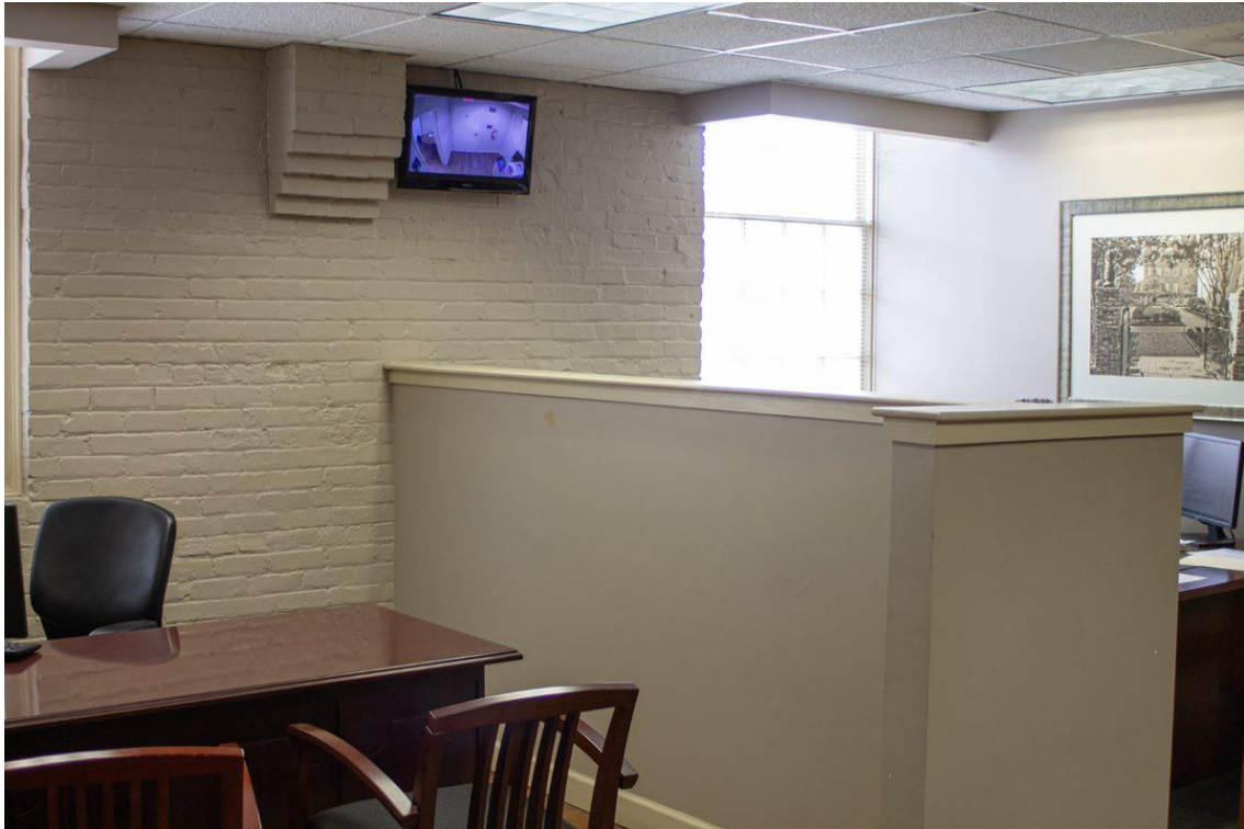
Photo 23 Southwest office detail. Note acoustic panel drop ceiling articulated to accommodate historic window height and corbeled brick terminus of second-story, narrow chimney originally used for coal-burning stoves.
