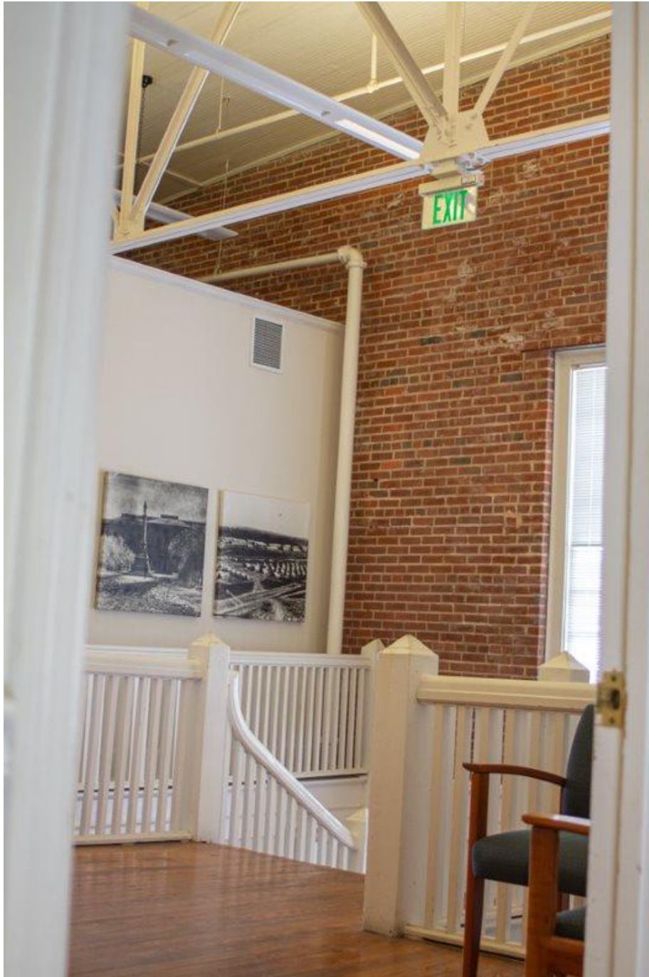
Photo 33 Third-story landing. Note original floor, exposed brick wall, balustrade, newel post and steel bow-truss details.
