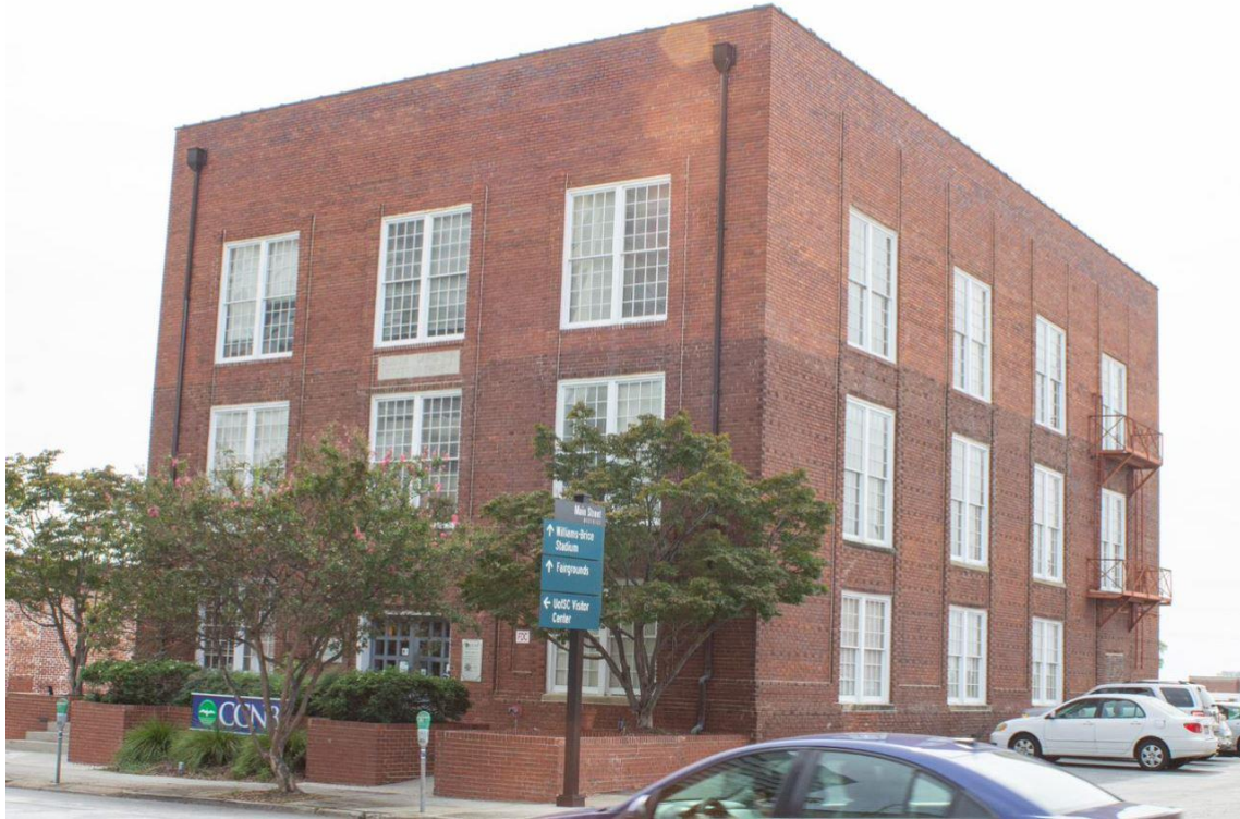
Photo 1 – Façade/east elevation & north elevation (northeast oblique view)
