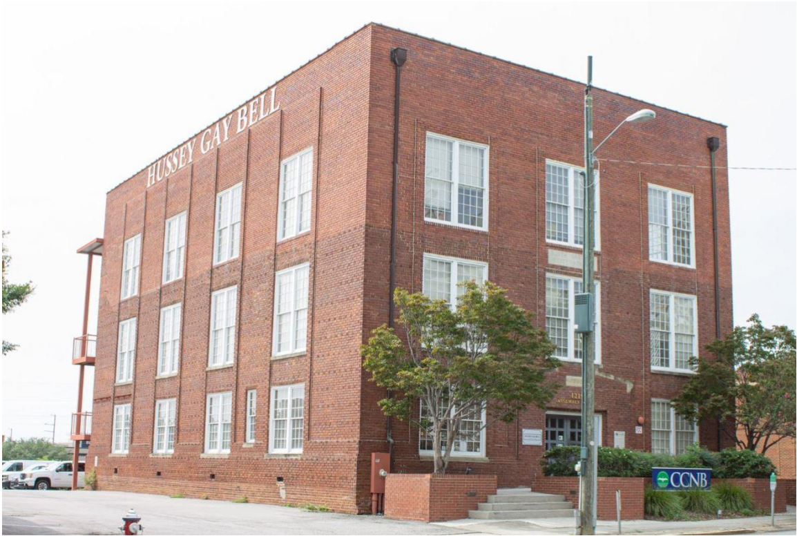
Photo 2 – Façade/east elevation & south elevation (southeast oblique view)
