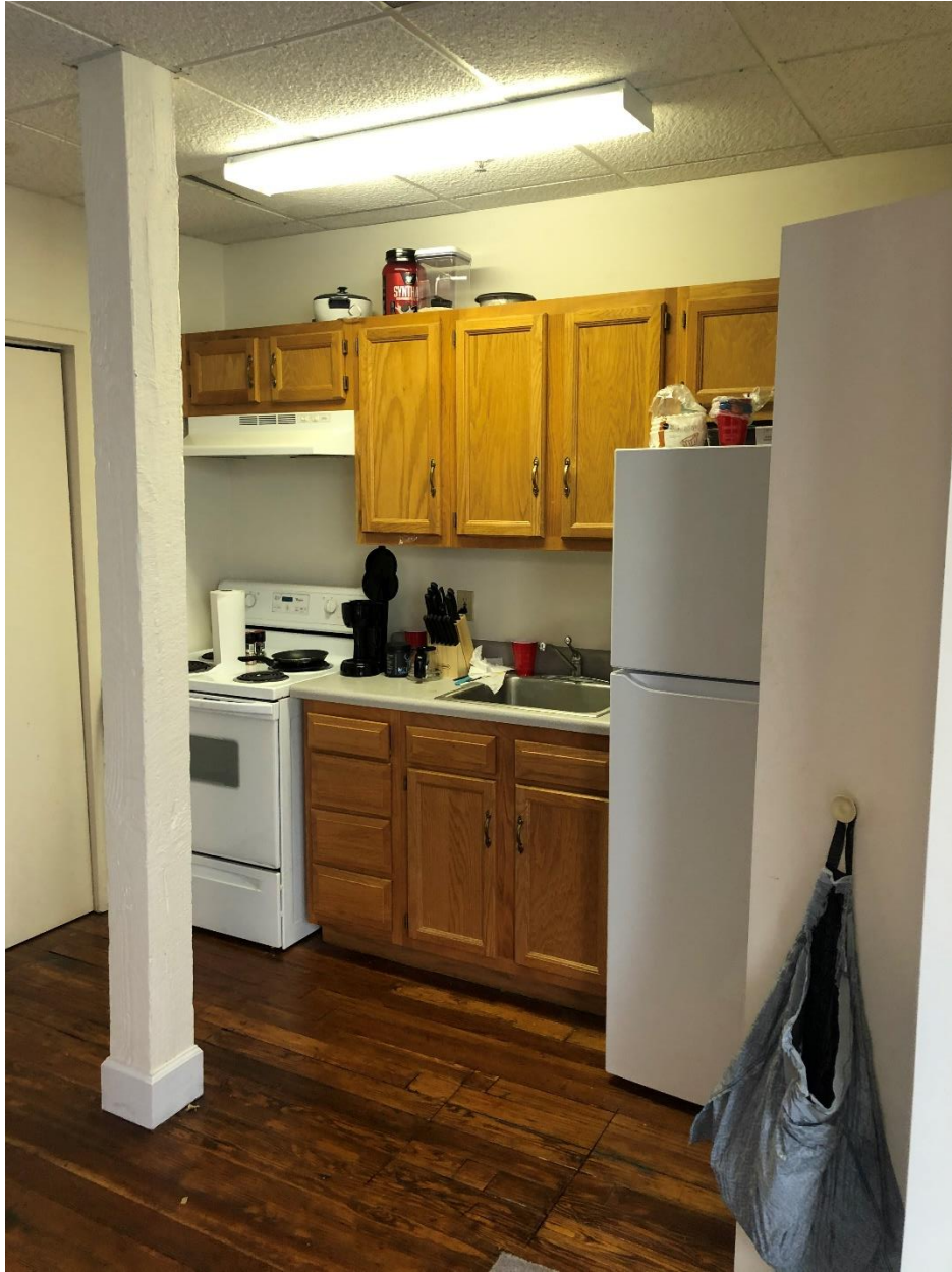
Photo 40 Southwest apartment detail. Note historic, rough-cut wood column.
