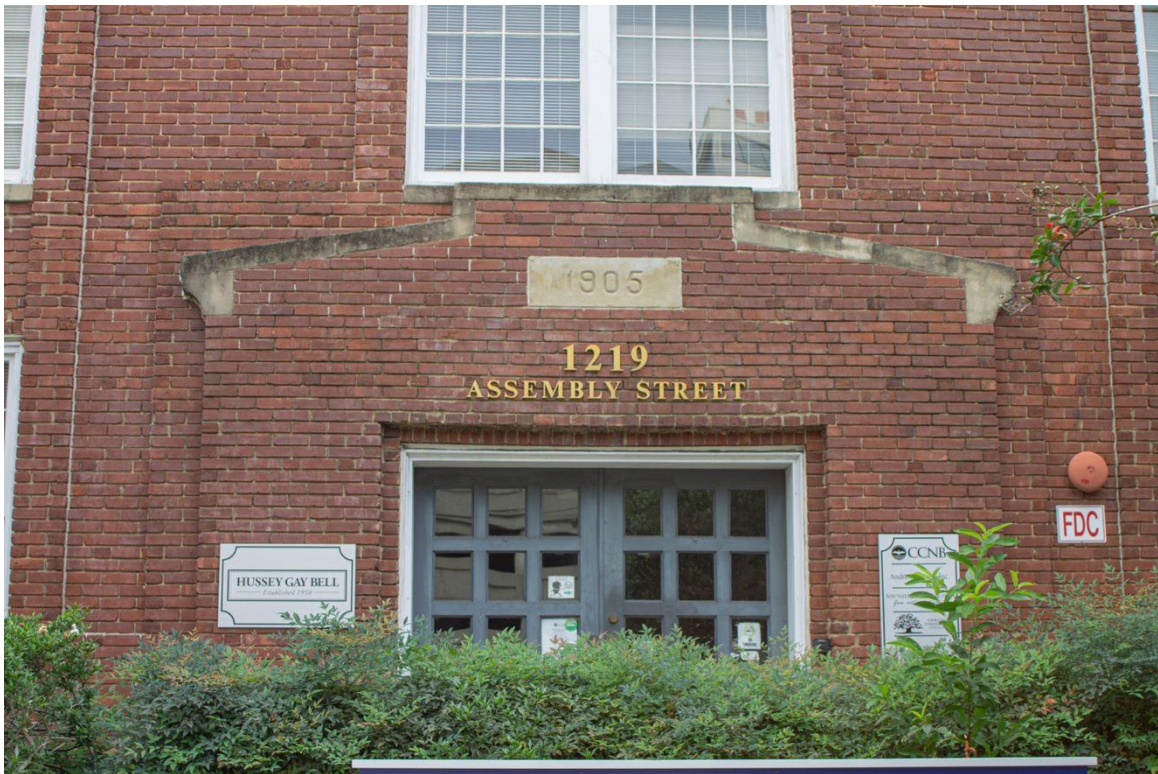
Photo 3 – Façade/East elevation (main entry detail view)
