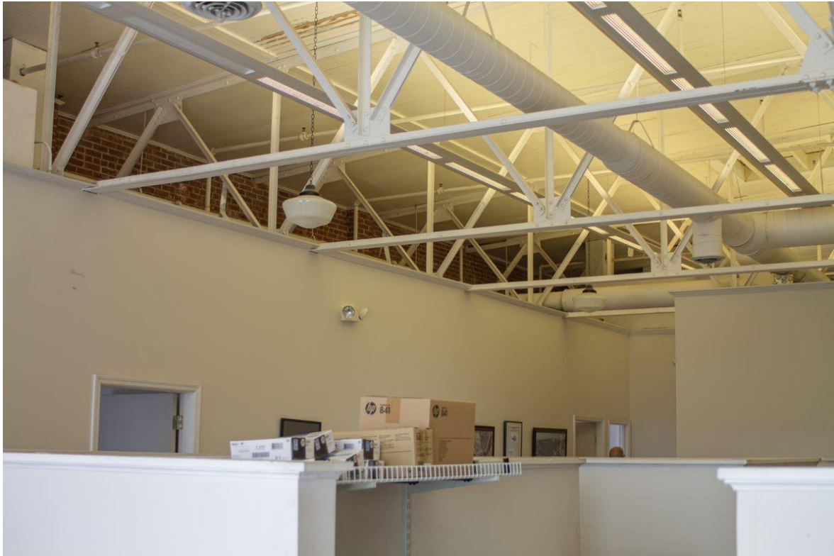
Photo 36 Third-story central office general conditions. Note steel bow truss details, exposed HVAC ductwork and historically inspired pendant lights.
