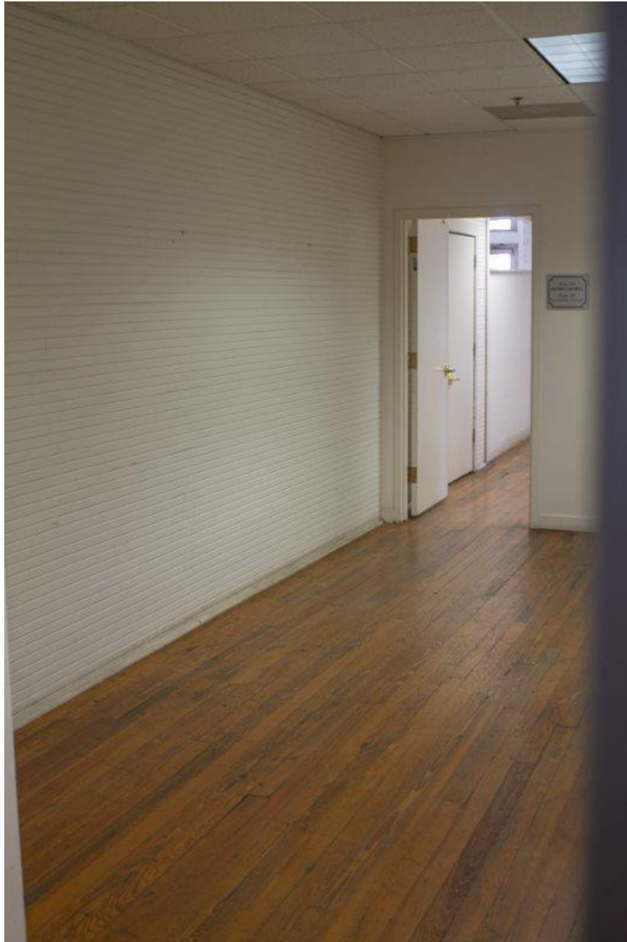
Photo 28 Second-story primary hallway. Note historic, vertically oriented, beadboard panel wall.
