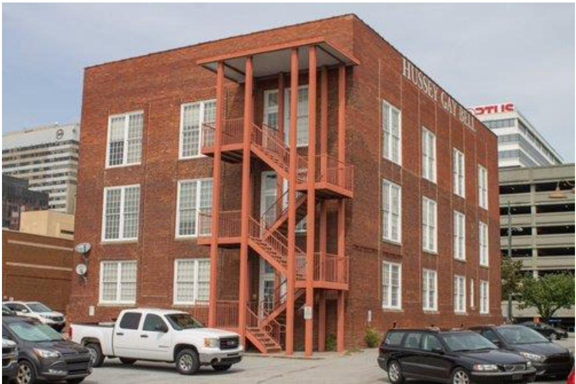
Photo 7 – West elevation & south elevation (southwest oblique view). Note visual vertical emphasis created by placing windows in one-half-depth brick butters/projection.
