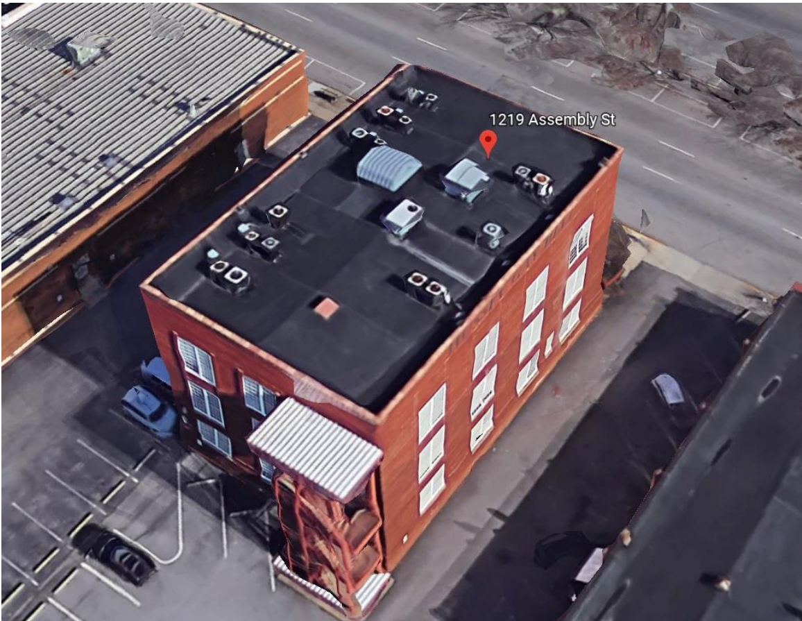
Photo 39 General roof conditions, looking northeast.
