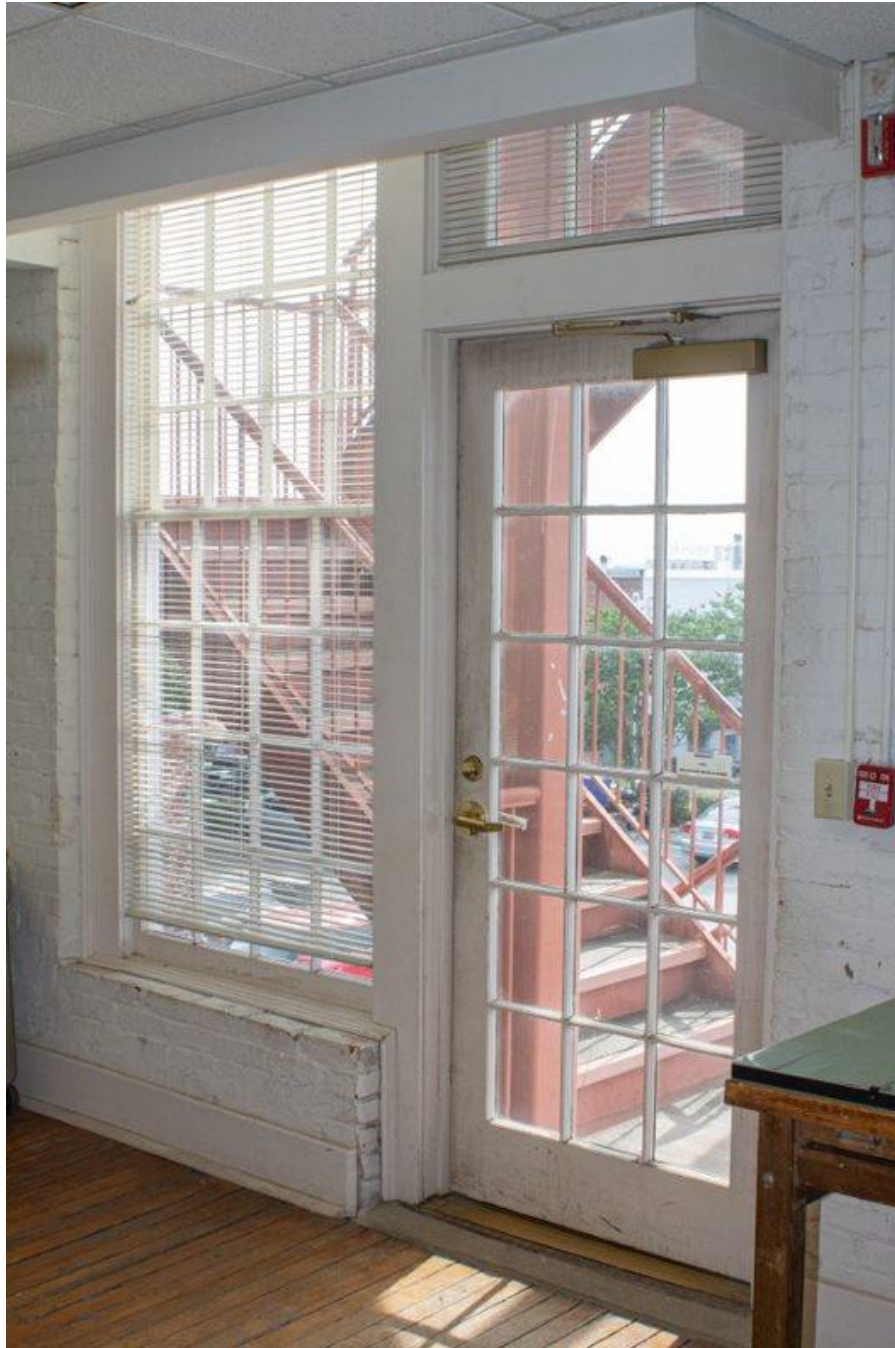
Photo 31 Second-story west office, looking west. Note exposed masonry wall and ca.-1998 rear stair entry/exit.
