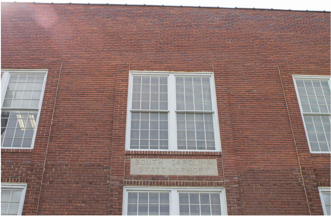
Photo 4 – Façade/East elevation (name plaque & brick transition detail view)
