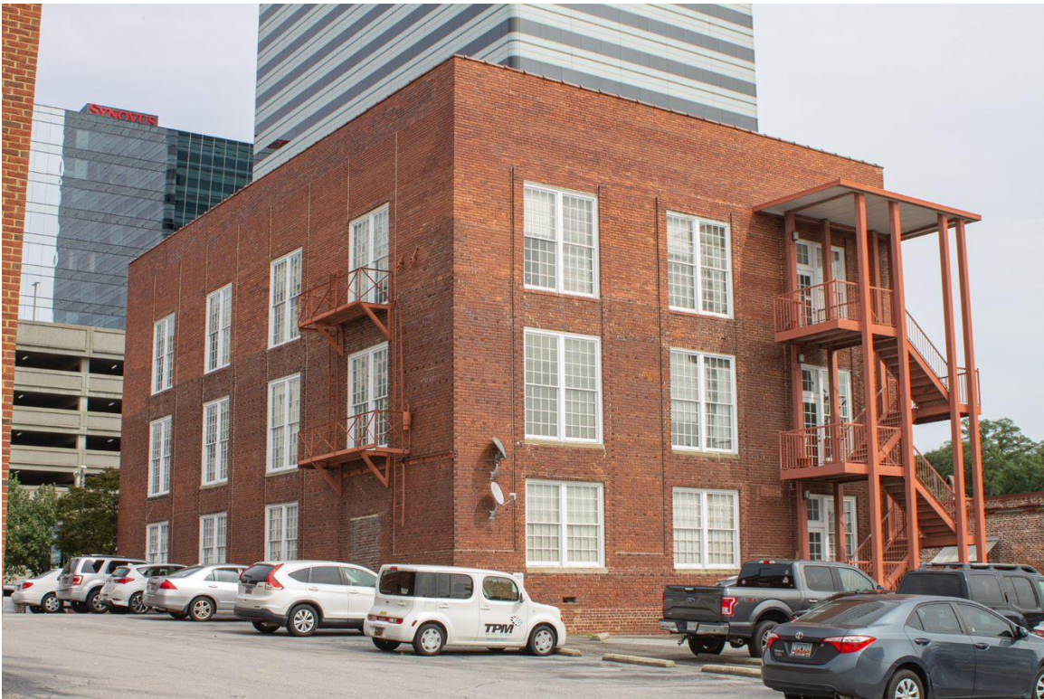
Photo 5 – North elevation & west elevation (northwest oblique view)
