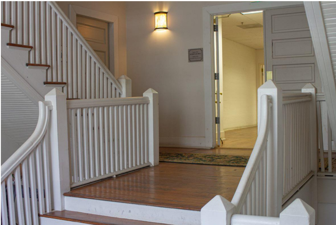
Photo 27 Second-story primary landing. Second-story landing. Note original hardwood floors and historic single and double doors.
