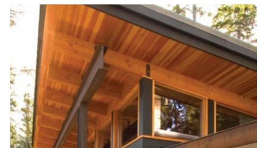
5. Stained Wood Soffit
