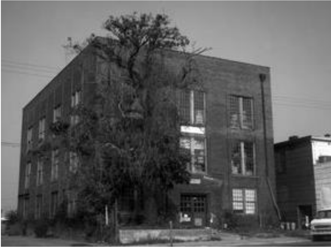
Photo 43 1219 Assembly Street, Pre-rehabilitation B&W Photograph of South Carolina State Armory Building
