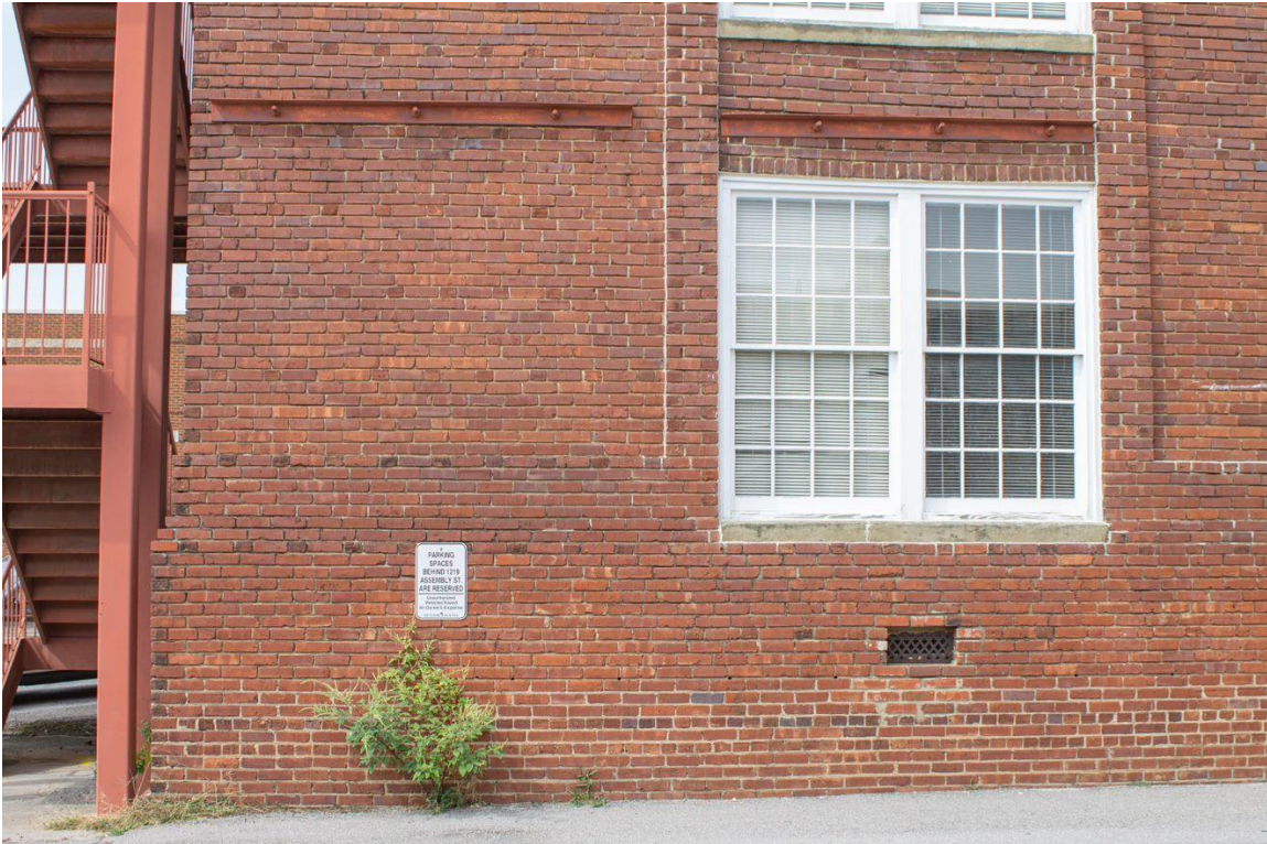
Photo 9 – South elevation detail. Note L-angle steel supplemental structural supports.
