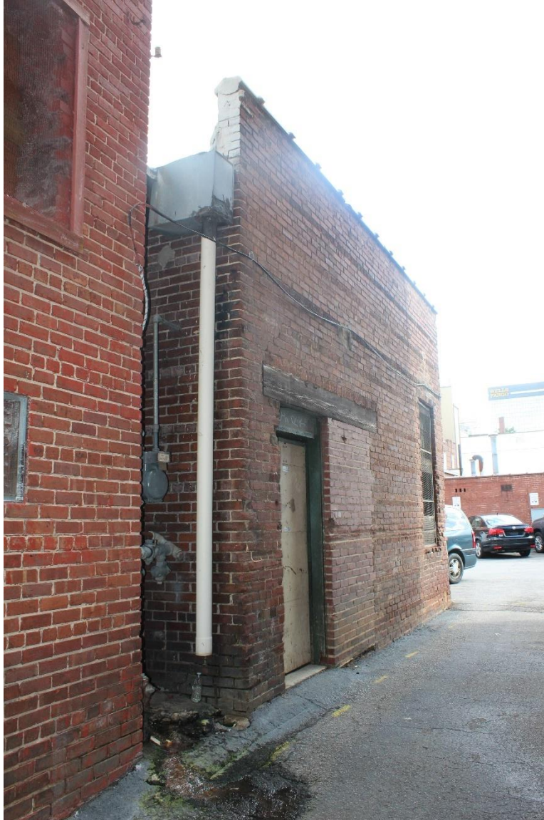
Photo 6 – West elevation looking south
