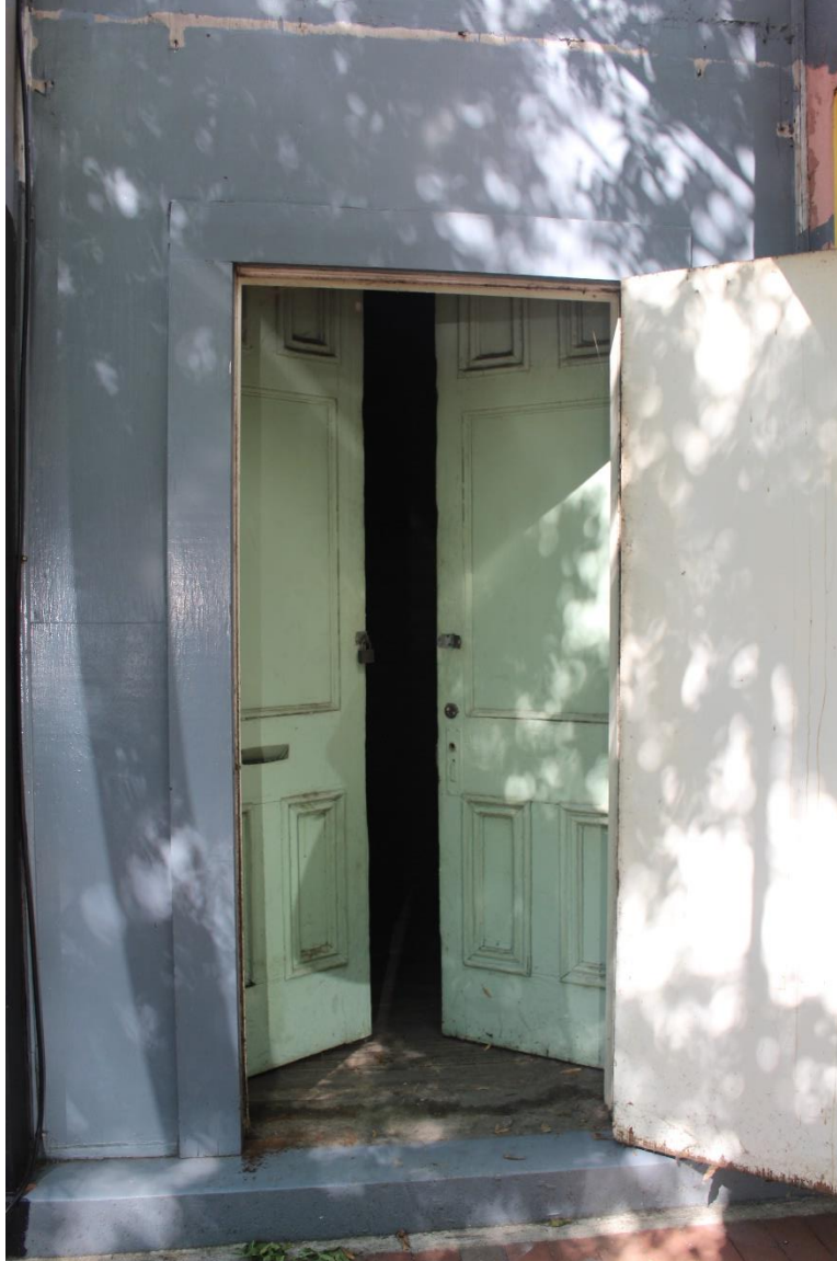
Photo 15 – Original doors to stairwell, east façade
