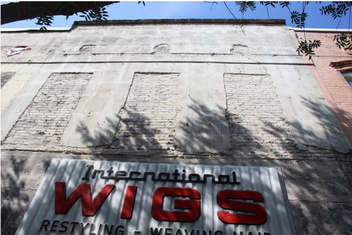
Photo 3 – East façade of 1643 Main Street
