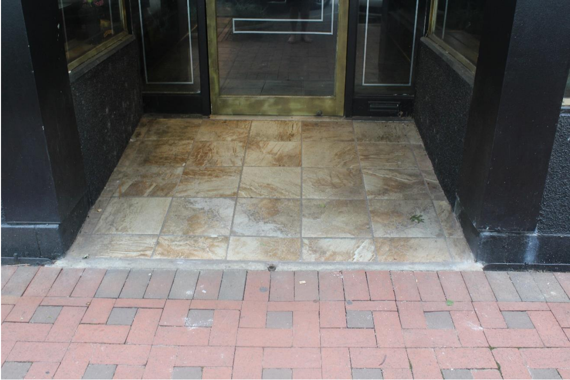
Photo 6 – Storefront entry tile, east façade of 1639 Main St. bay
