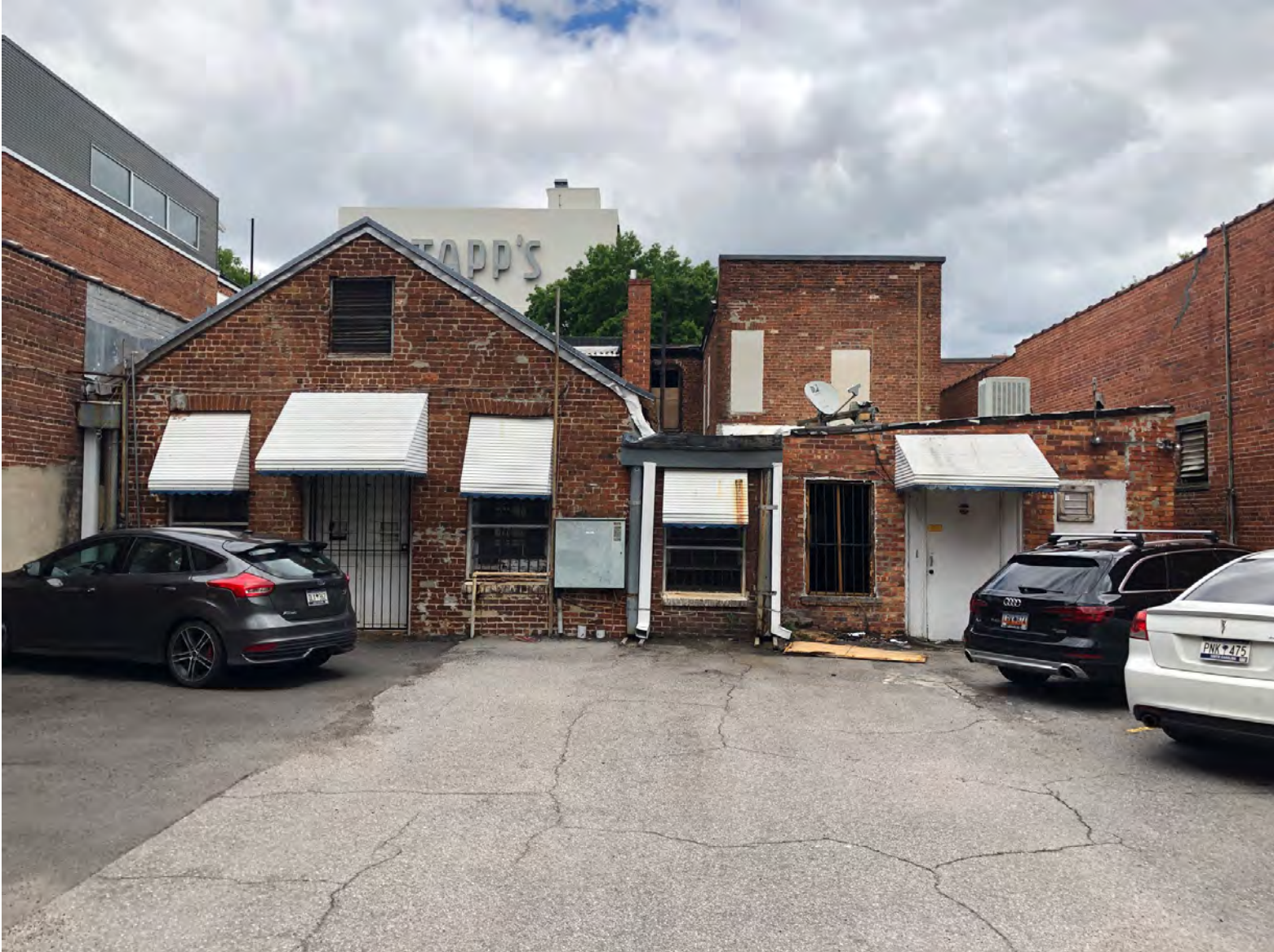
EXISTING CONDITIONS PHOTO - REAR PARKING LOT
