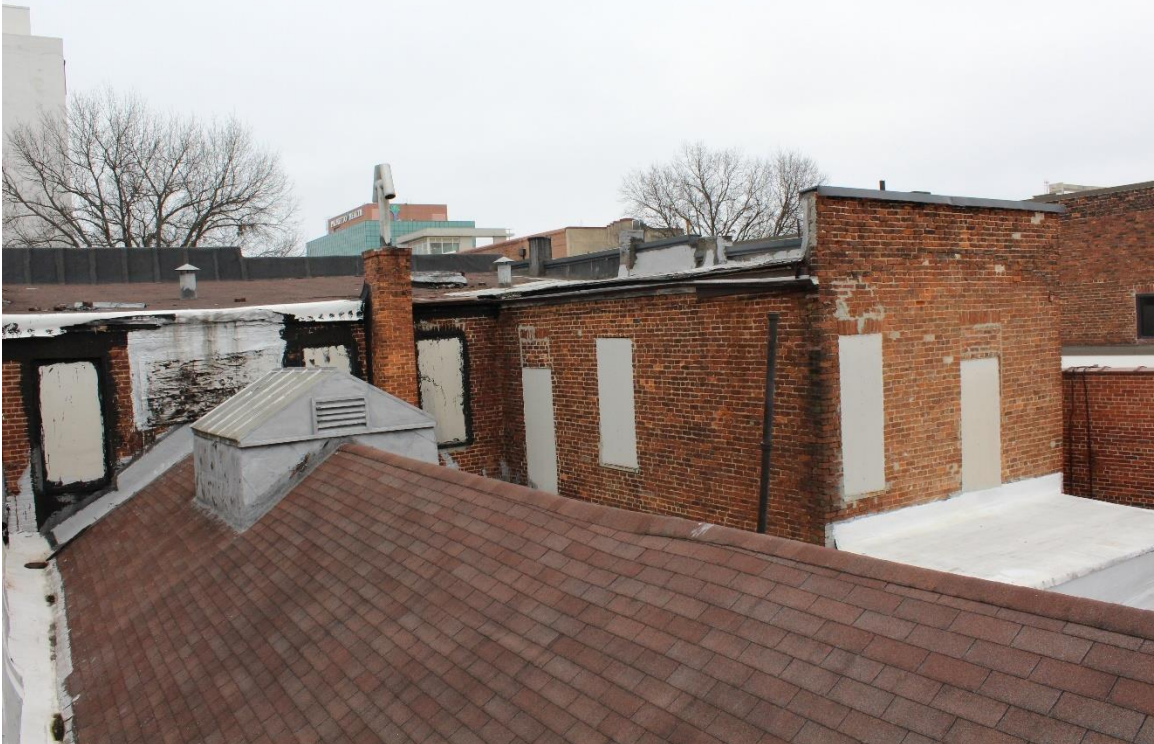
Photo 14 – Second floor northwest oblique
