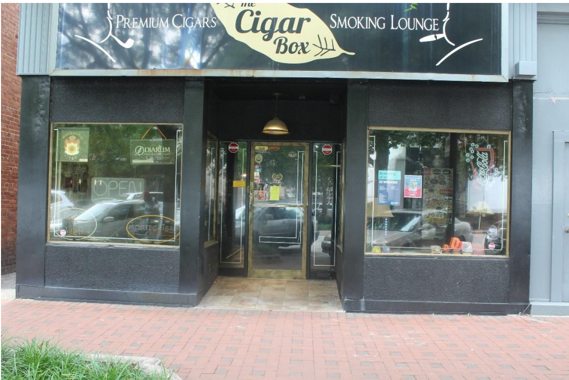
Photo 5 – 1639 Main Street storefront
