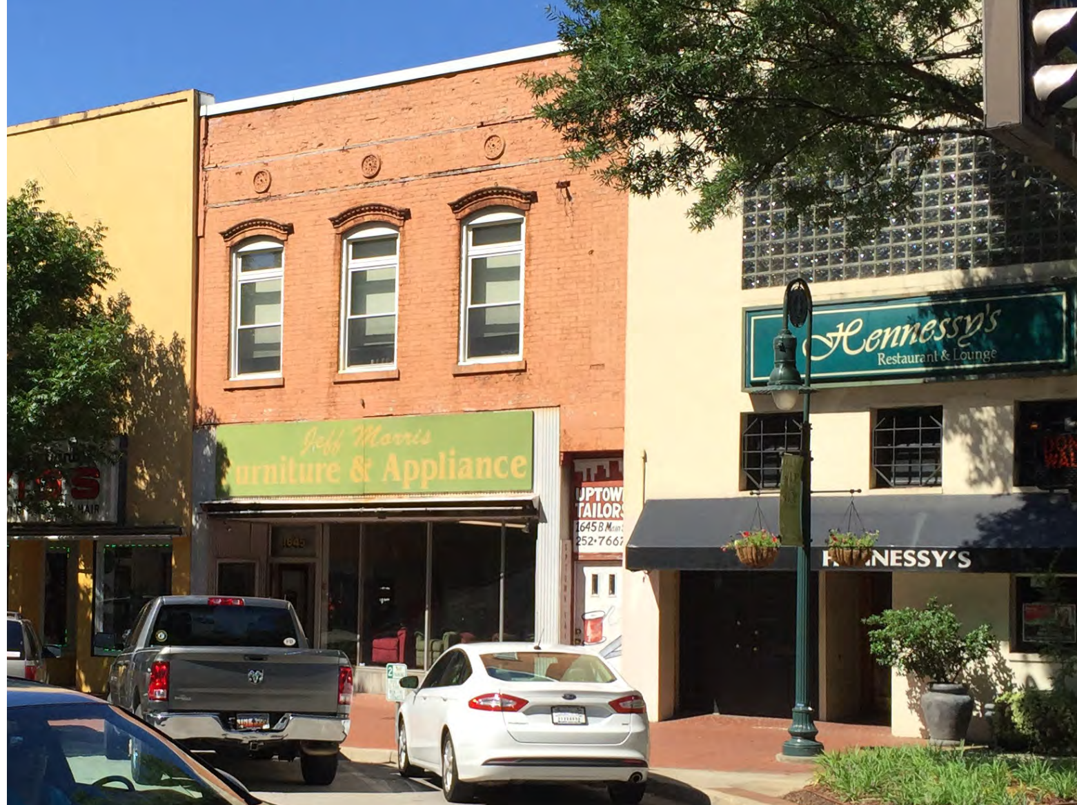
EXISTING CONDITIONS PHOTO - 1645 MAIN STREET
