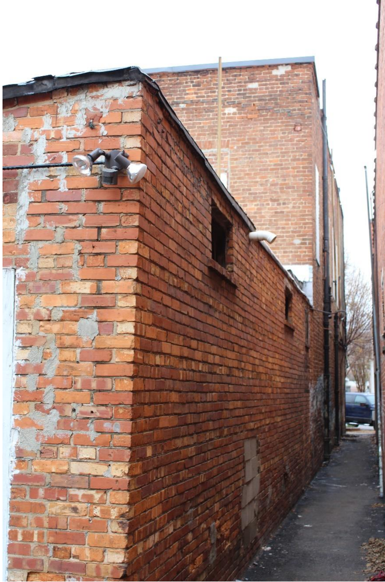
Photo 10 – South elevation looking east
