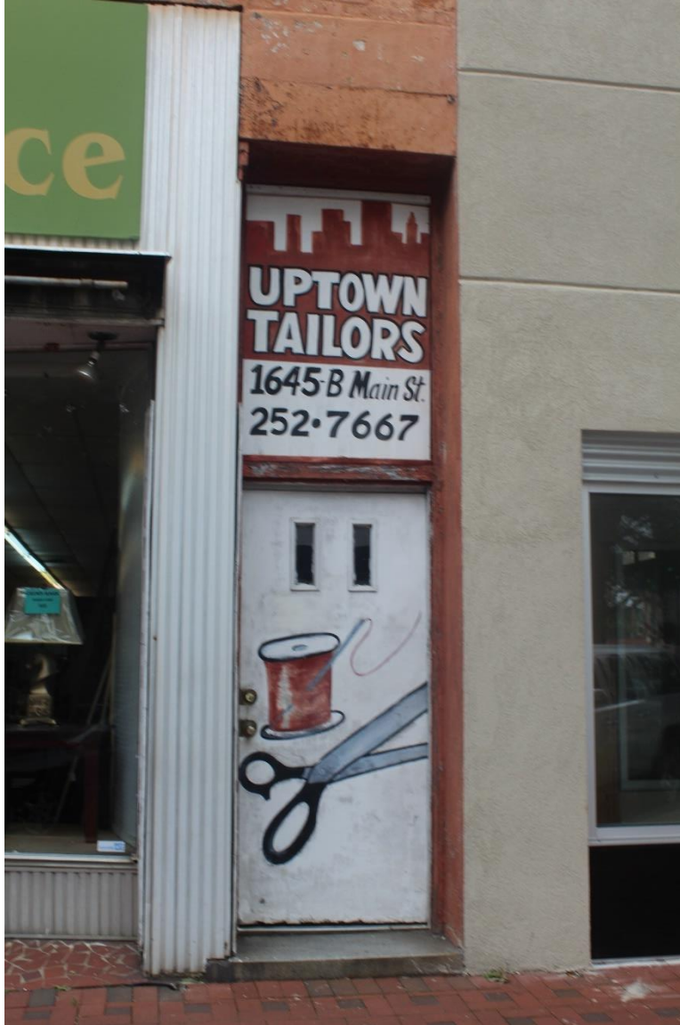
Photo 4 – Stairwell door, north end of west façade
