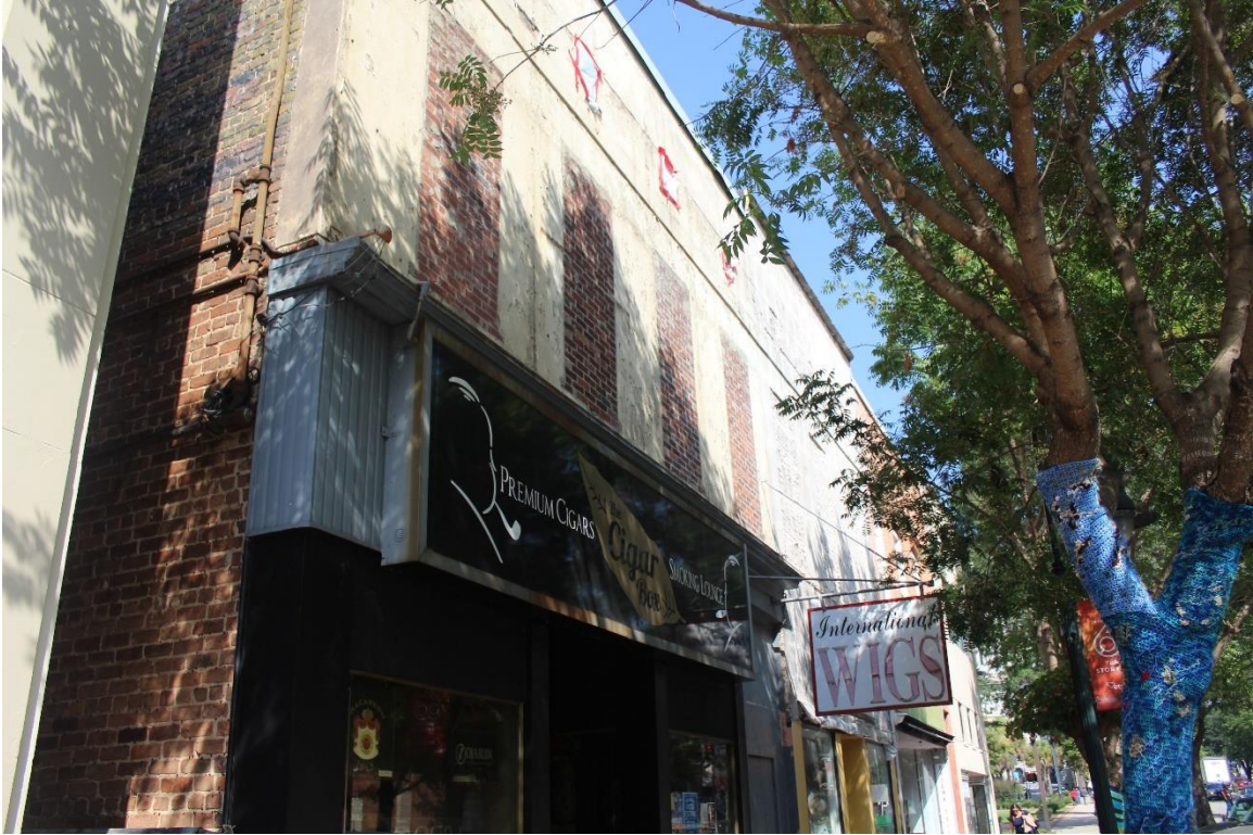
Photo 2 – East façade looking north
