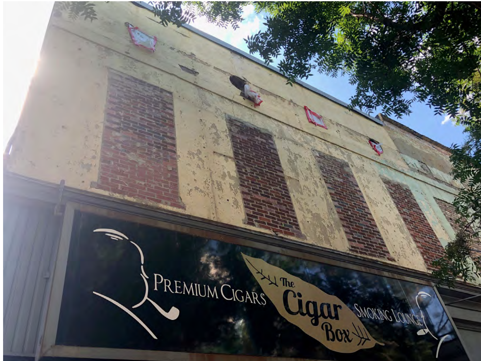
EXISTING CONDITIONS PHOTO - 1639 MAIN STREET
