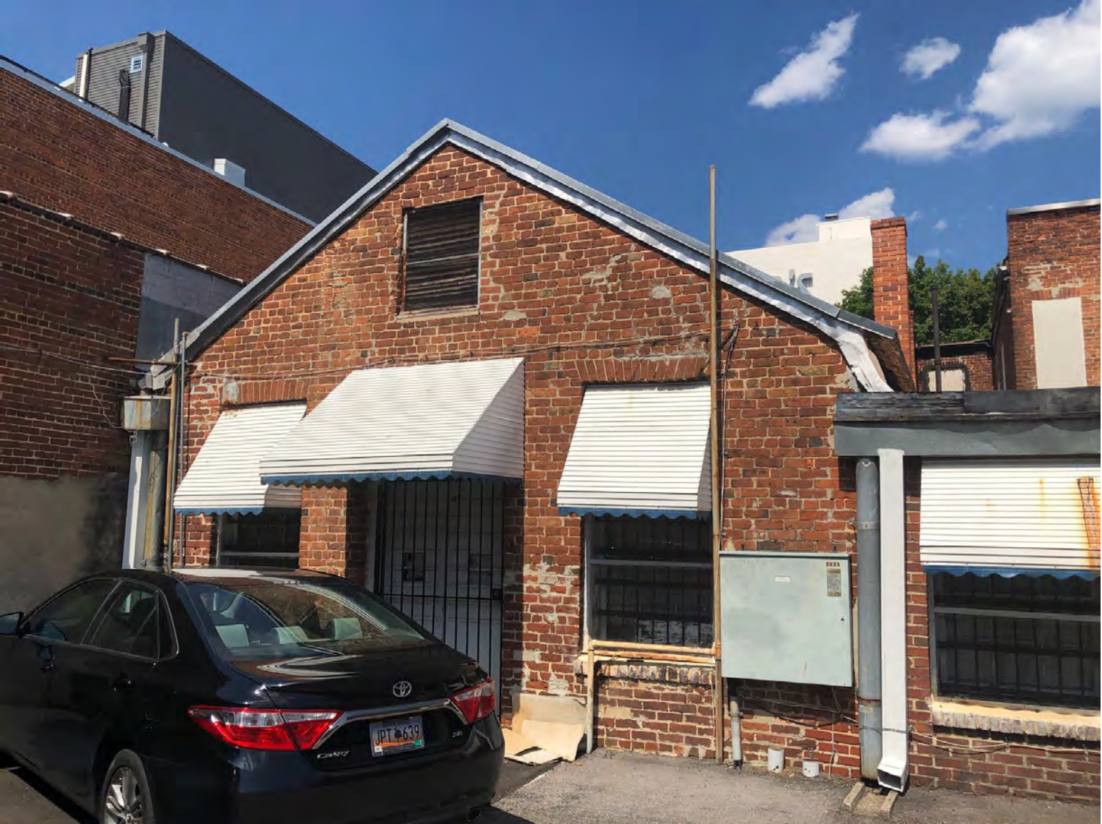
EXISTING CONDITIONS PHOTO - REAR PARKING LOT
