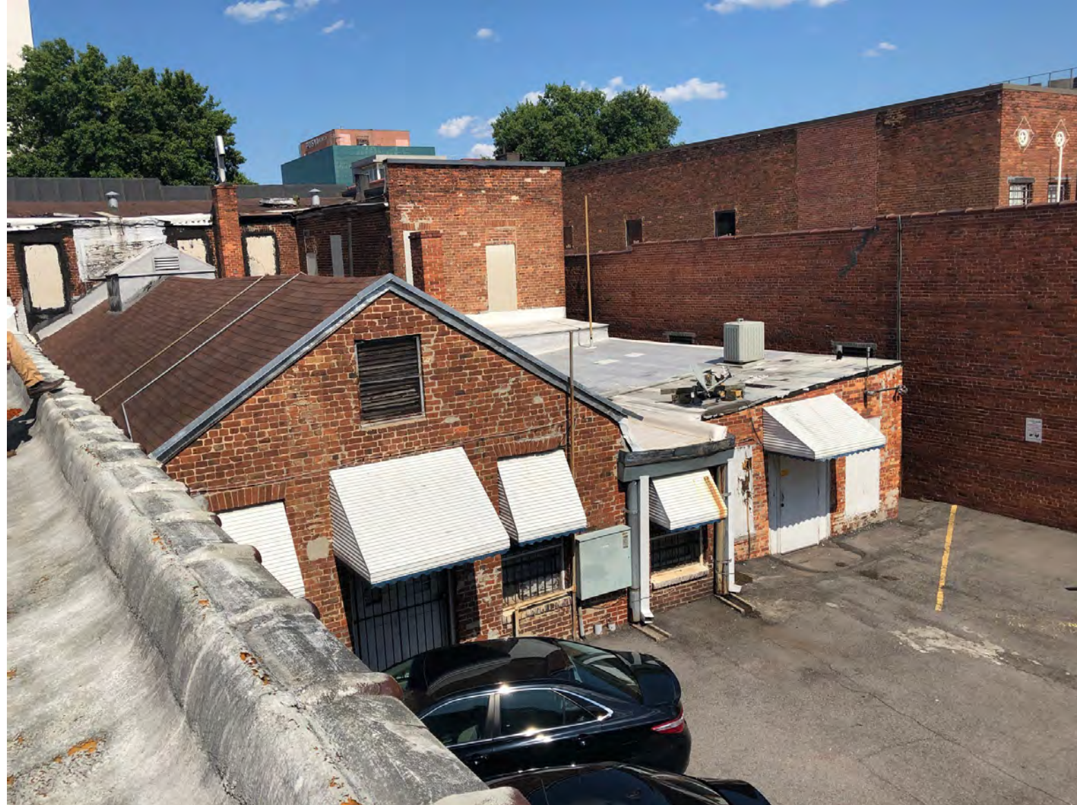
EXISTING CONDITIONS PHOTO - REAR PARKING LOT
