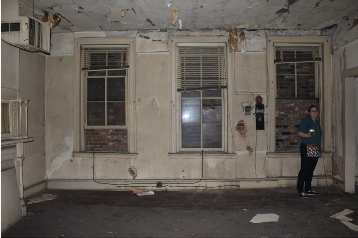
Photo 33 – Northeast corner room with original windows, second floor, looking east
