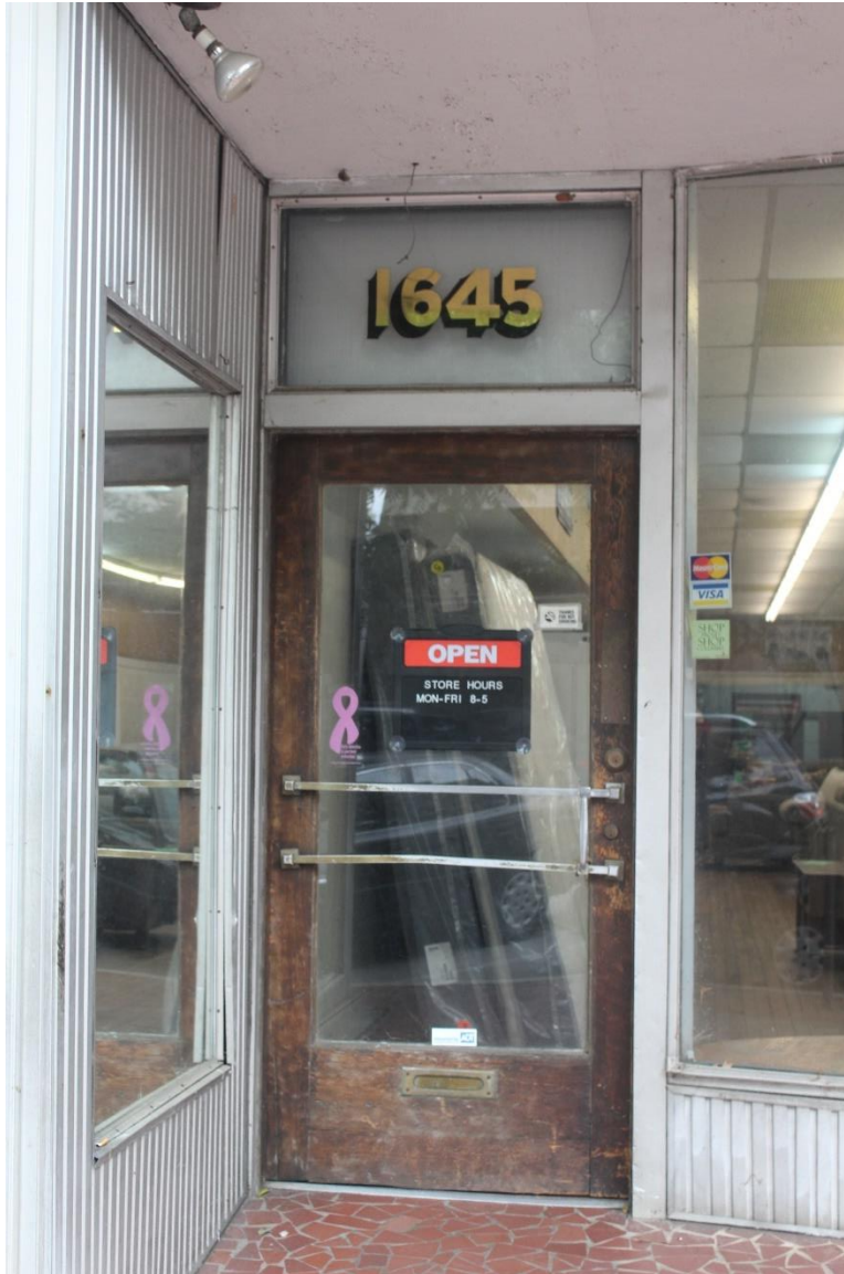
Photo 5 – Storefront door, south end of east façade
