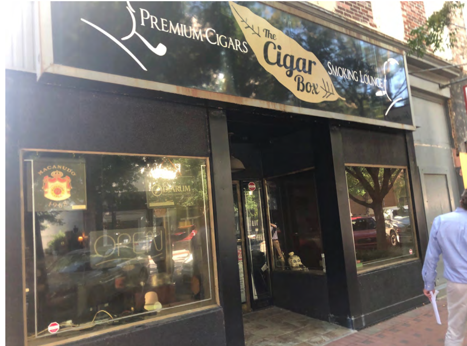
EXISTING CONDITIONS PHOTO - 1639 MAIN STREET
