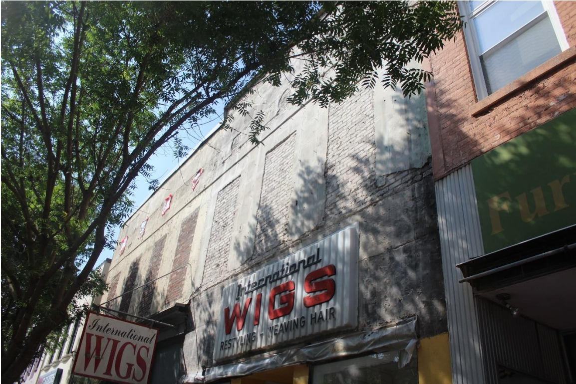
Photo 1 – East façade looking south
