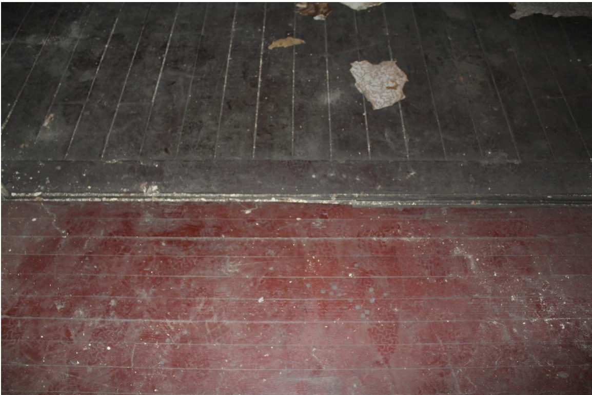
Photo 34 – Differing floors between northern rooms
