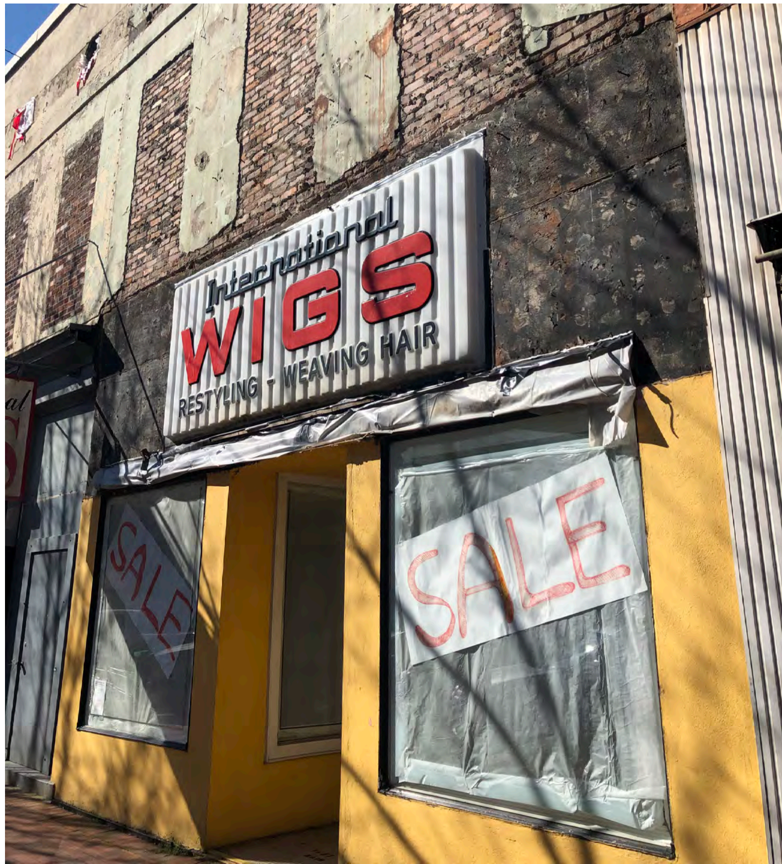
EXISTING CONDITIONS PHOTO - 1643 MAIN STREET
