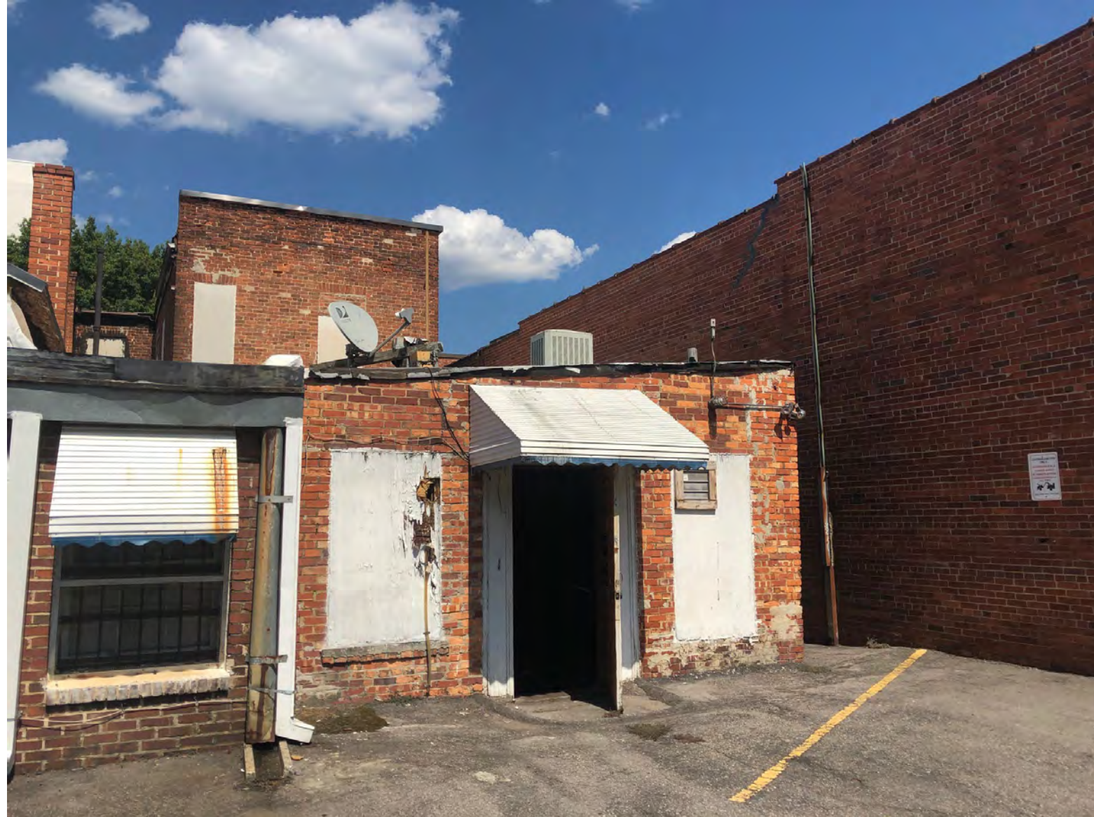
EXISTING CONDITIONS PHOTO - REAR PARKING LOT
