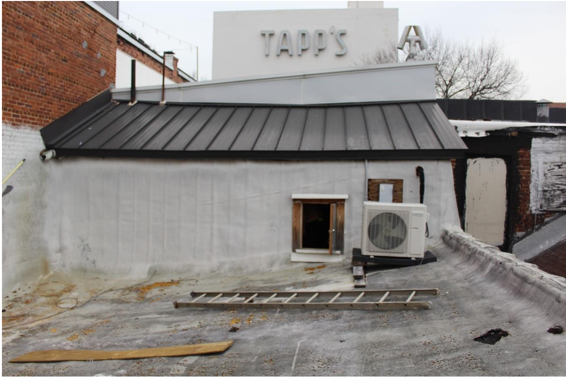
Photo 9 – Second floor roof, looking east
