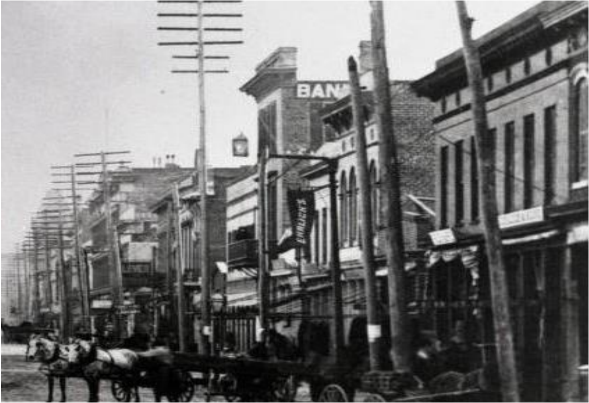
Photo 33 – Arched window and window hood at far right, c.1895 Courtesy of Walter Blanchard Collection
