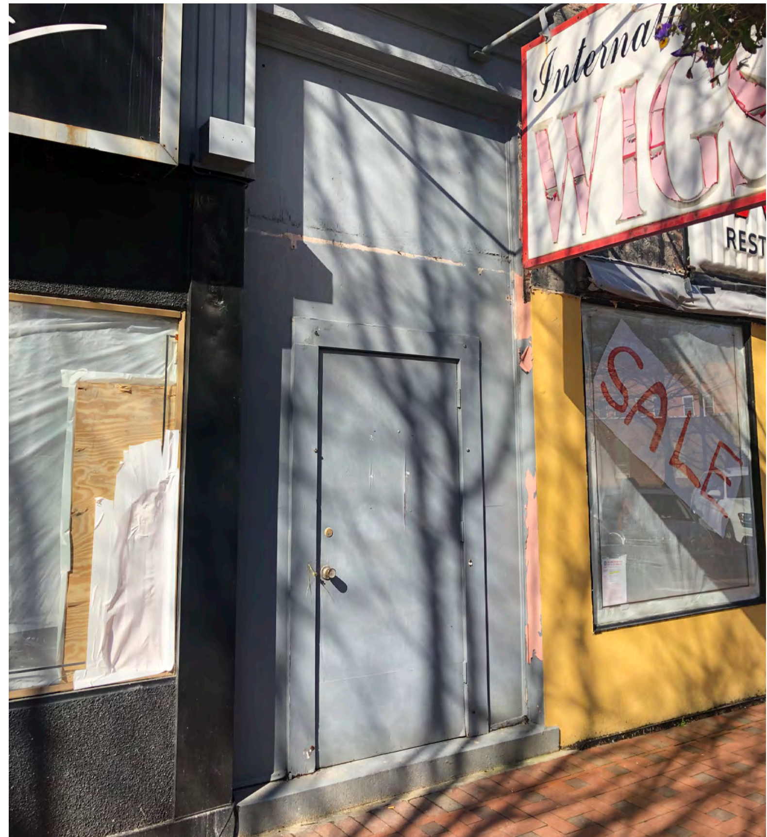
EXISTING CONDITIONS PHOTO - 1643 MAIN STREET
