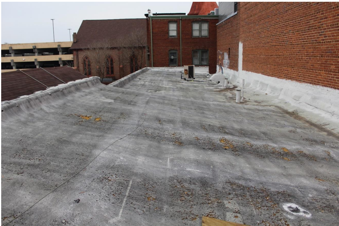
Photo 10 – Roof of one-story addition, looking west
