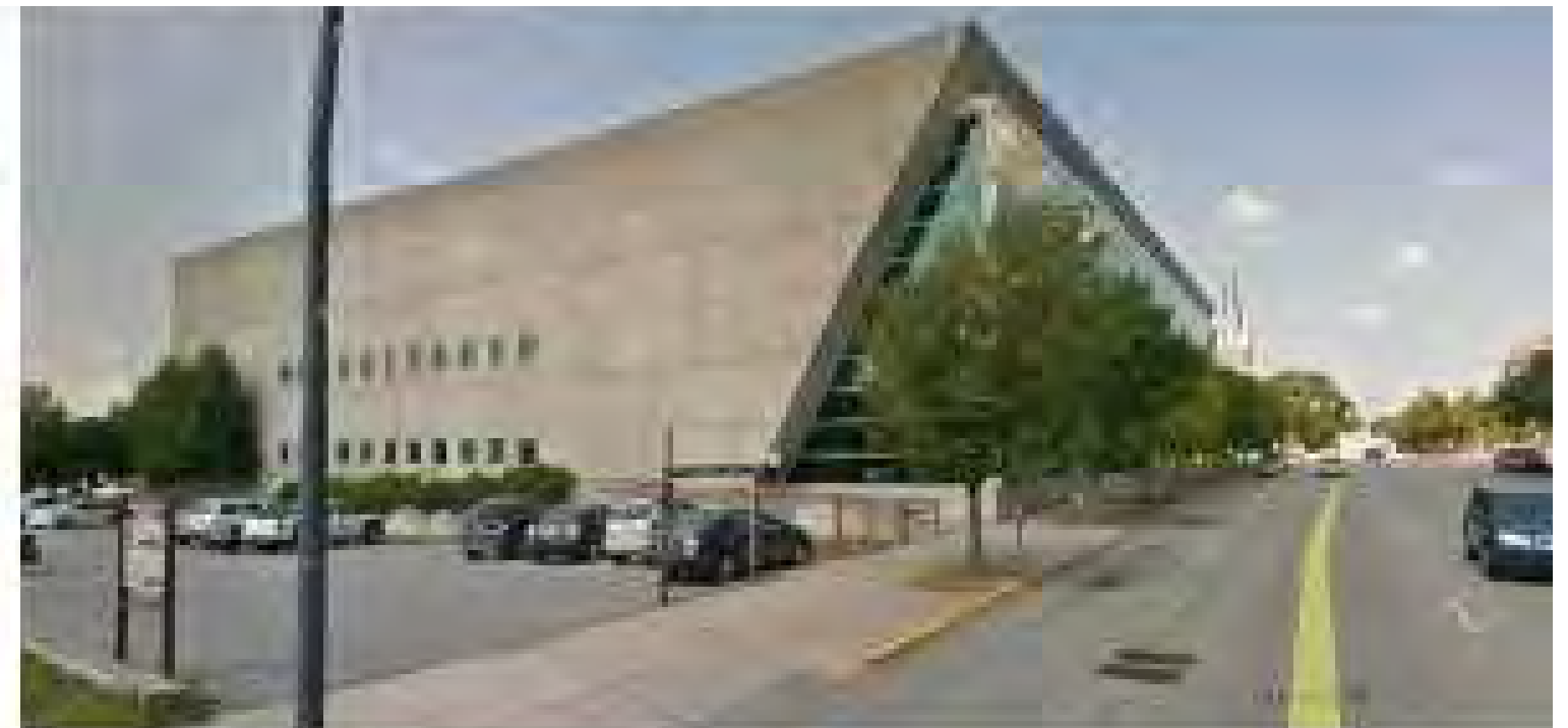
VIEW OF SITE FROM ASSEMBLY ST. LOOKING WEST
