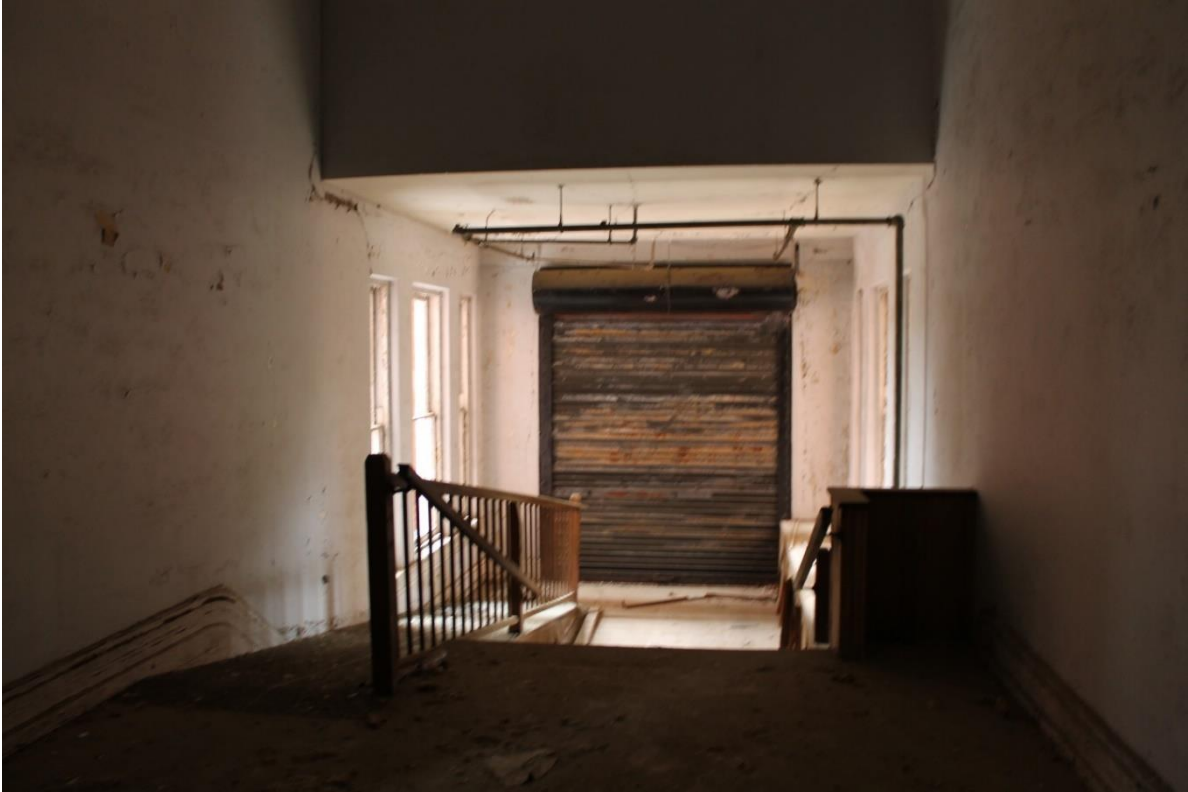
33. Center block, hyphen to southern wing, view to the south
