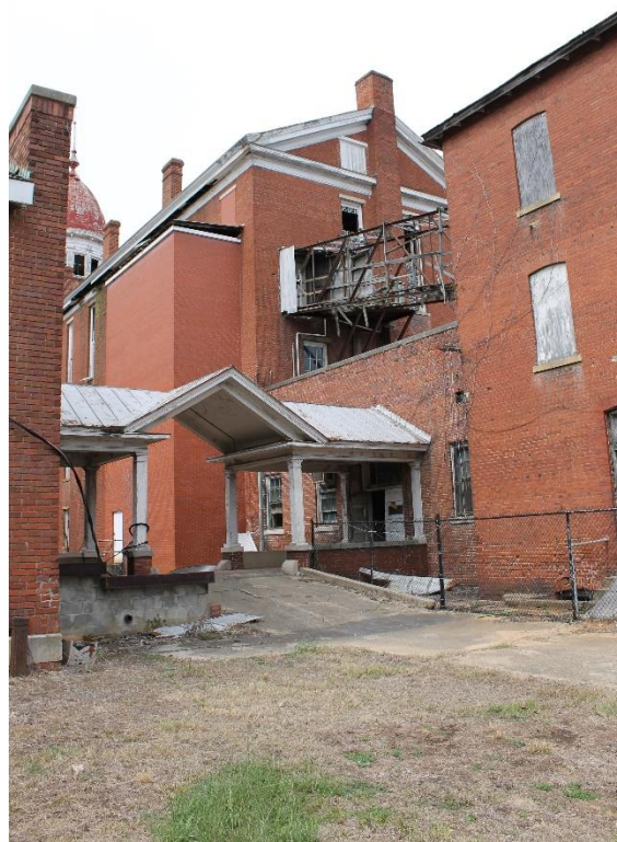
18. Center block – rear wing, view to the northwest
