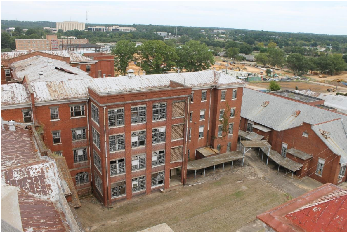
28. Northern east/west block and women's dining hall, view to the northeast
