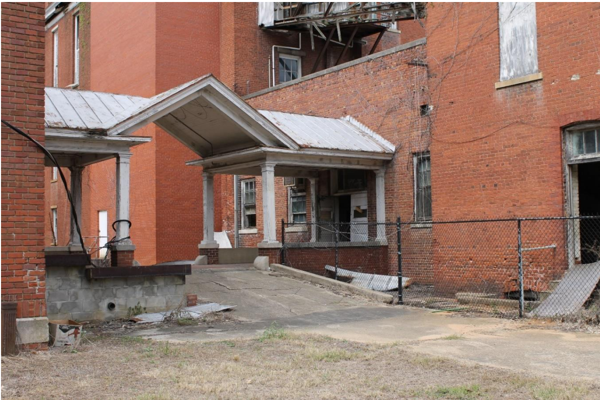
72. Men's dining hall hyphen to center block, view to the northwest
