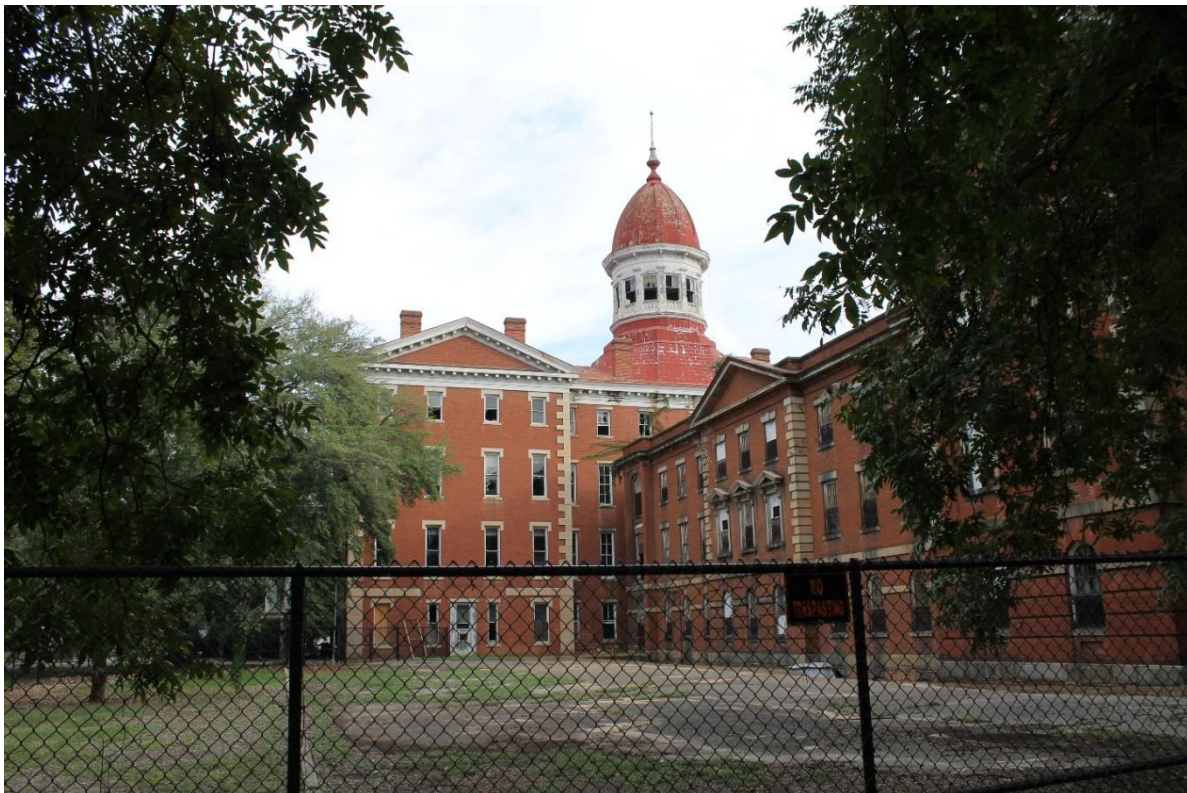
8. Center section and first southern north/south wing, view to the northeast
