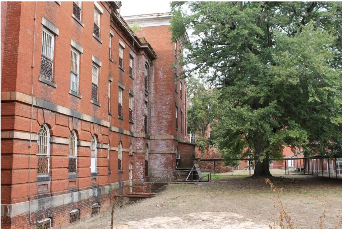
14. Rear of southernmost north/south wing and middle east/west block, view to the north
