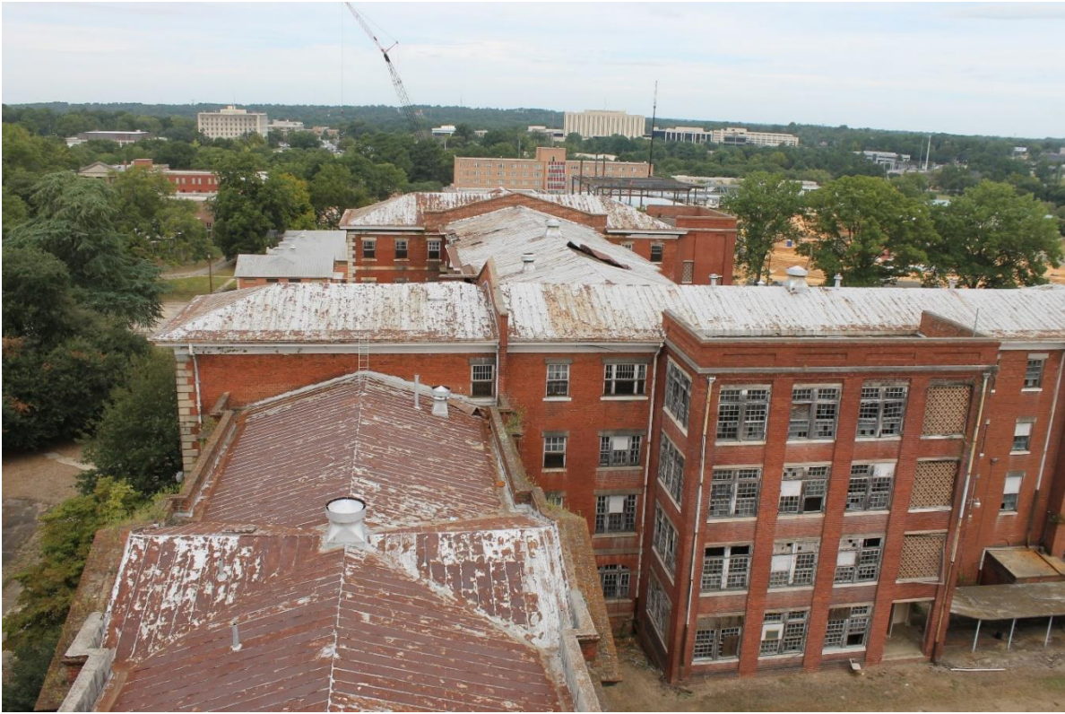
27. Roof, northern wings and east/west blocks, view to the north
