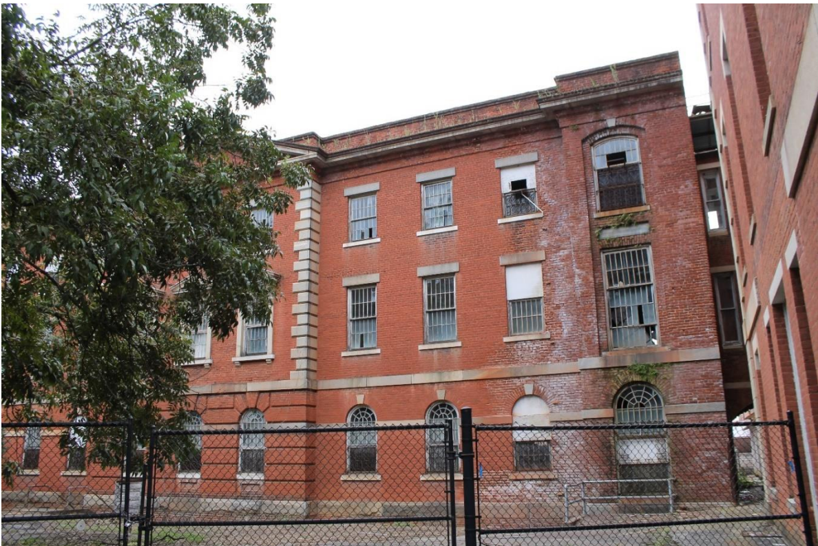
2. First northern north/south wing, view to the east
