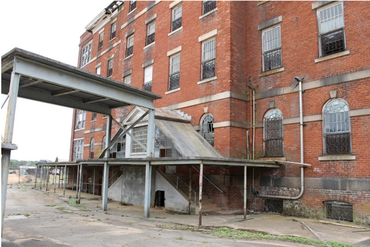
7. North side of northern terminal east/west block, view to the southeast
