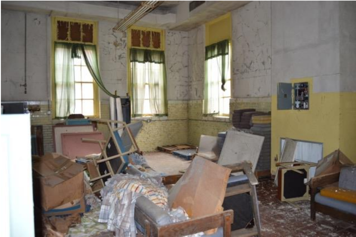
79. Men's dining hall interior
