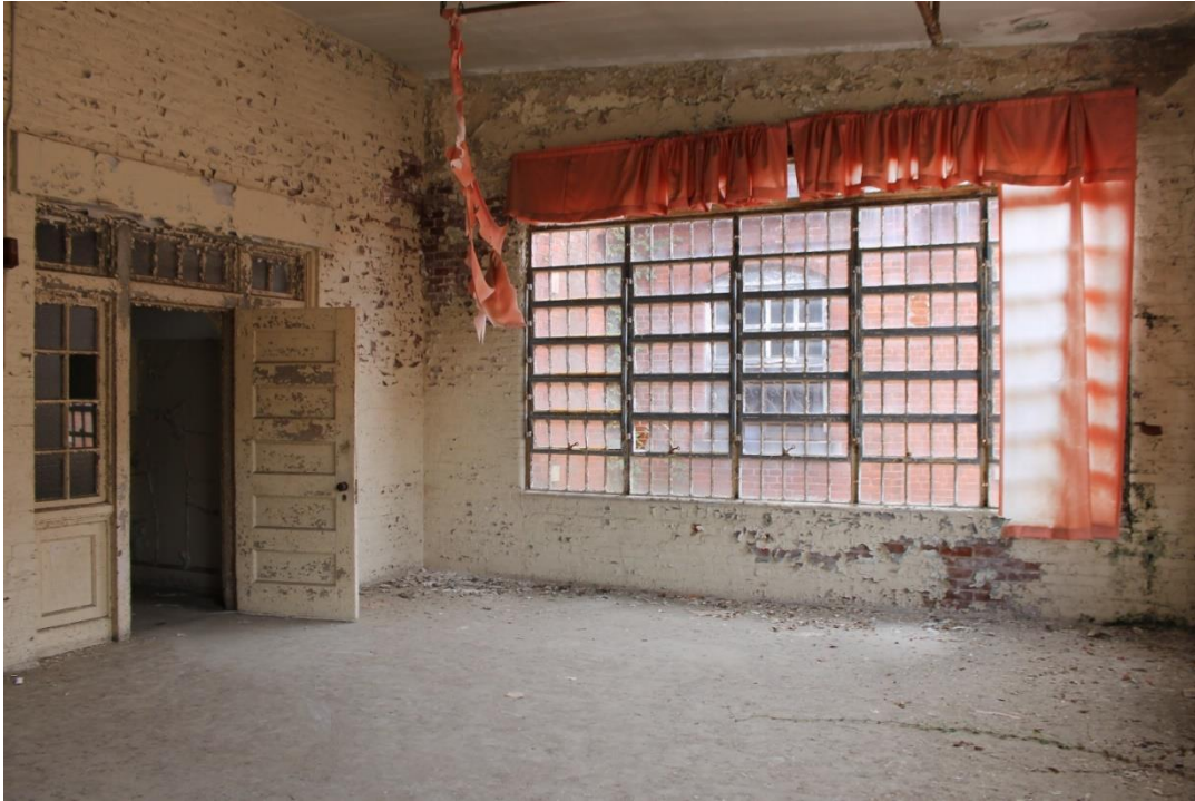
61. Southern section, sunroom addition, view to the northwest
