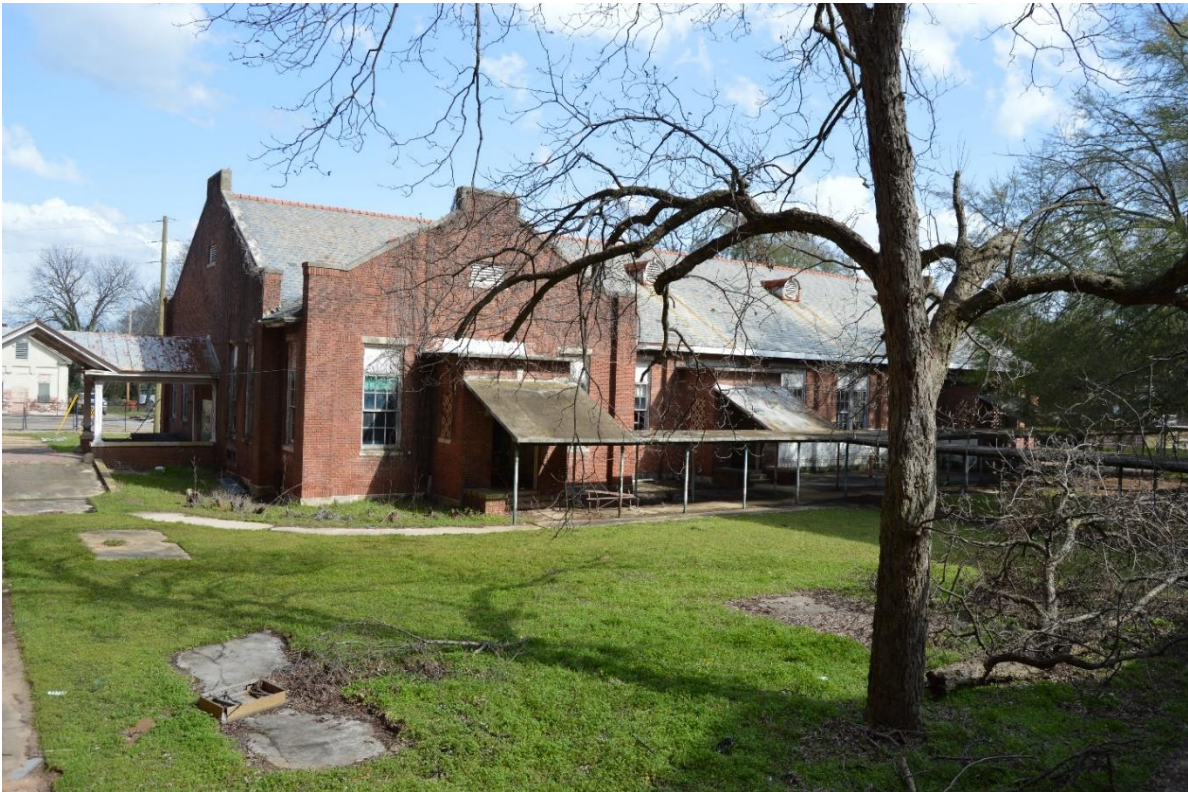
73. Men's dining hall, front and north end, view to the east
