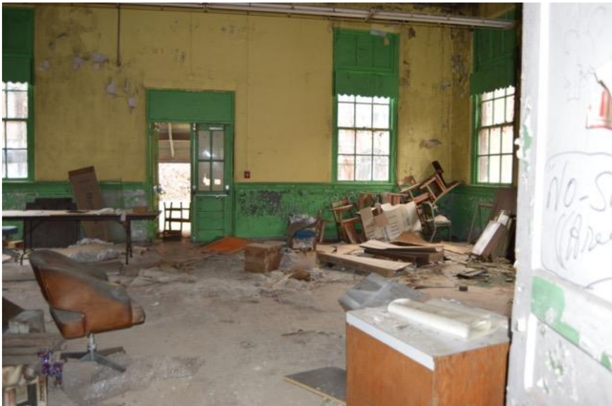
78. Men's dining hall interior
