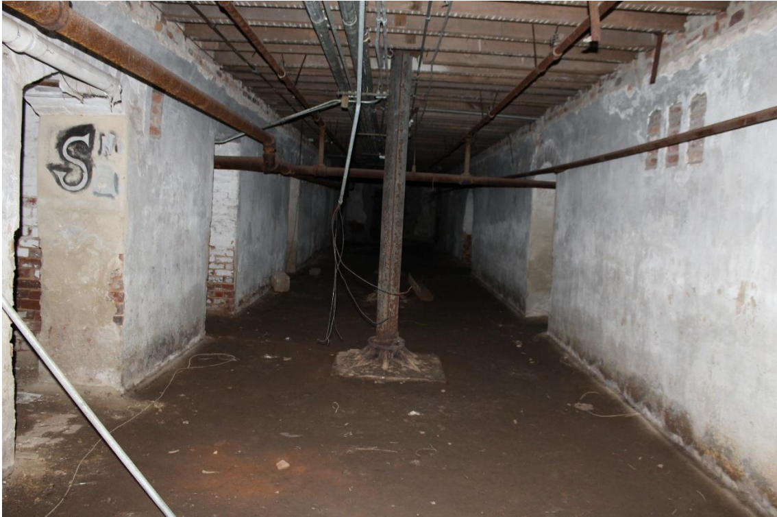
65. Basement, view to the south
