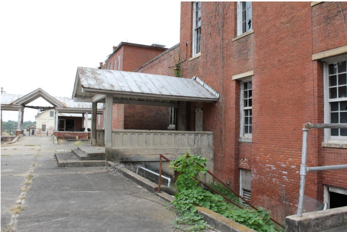
20. Porches on northern side of center block, view to the east
