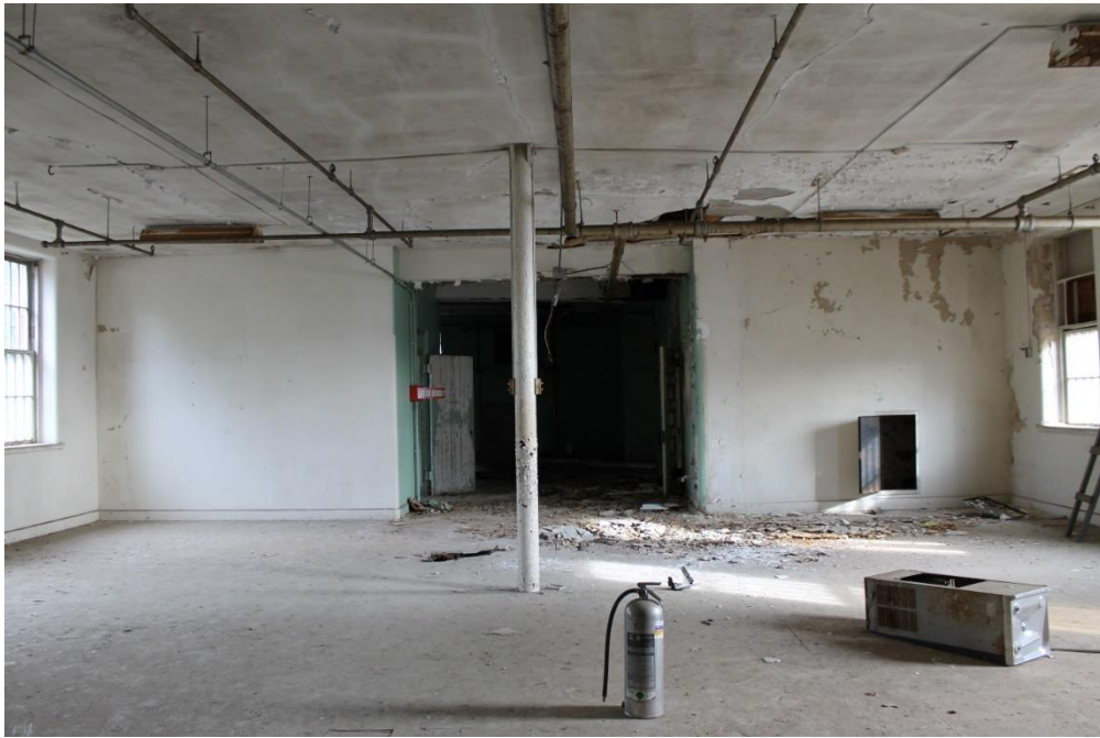
45. Northern wing, 2 nd floor, 1915 ward, view to the north
