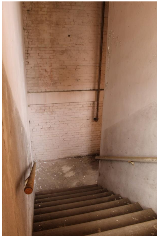
64. Stairs in sunroom addition
