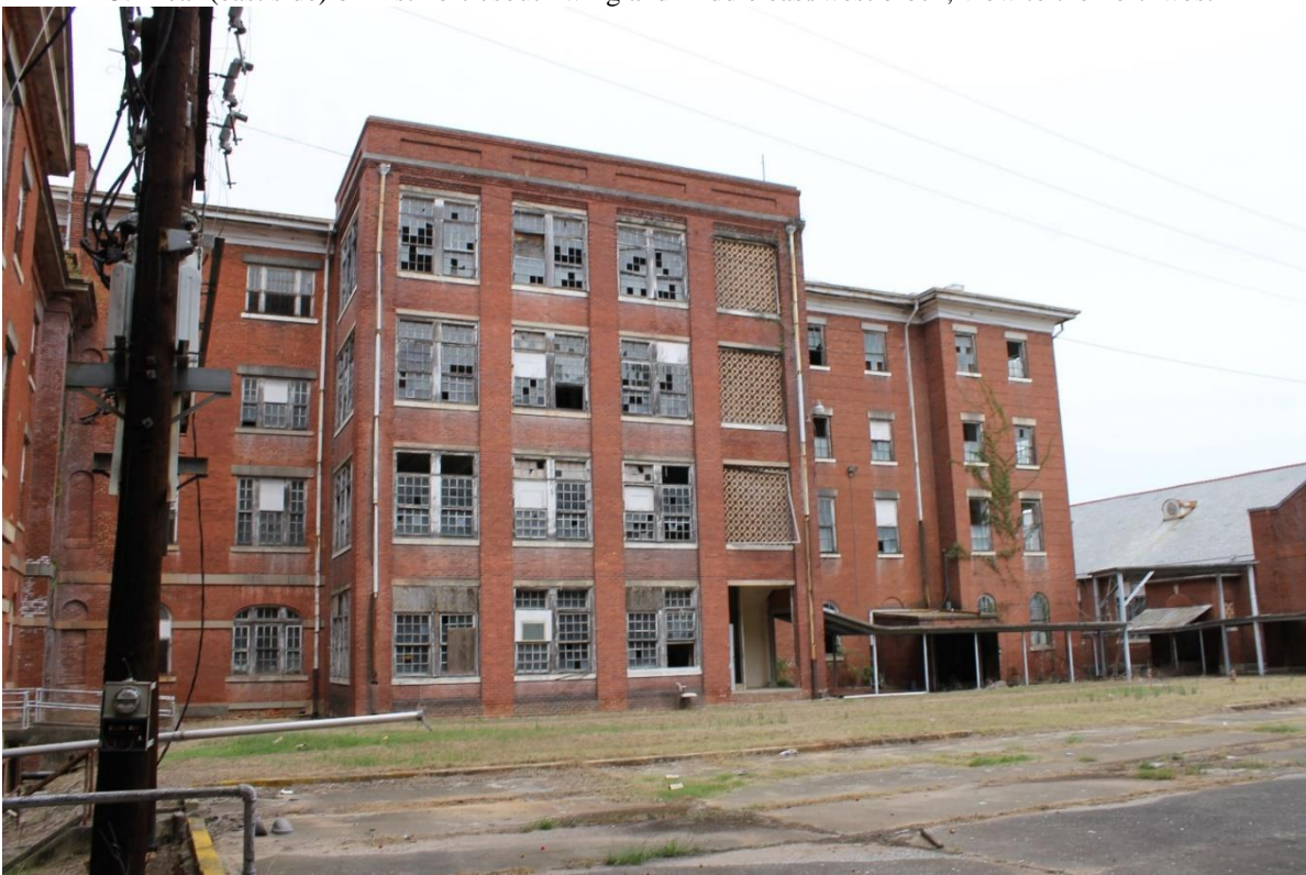
24. Southern side of middle east/west block, view to the northeast
