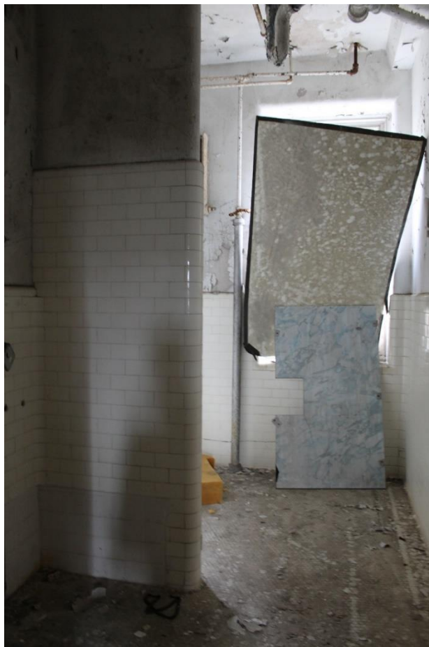
46. Northern wing, bathroom, view to the west
