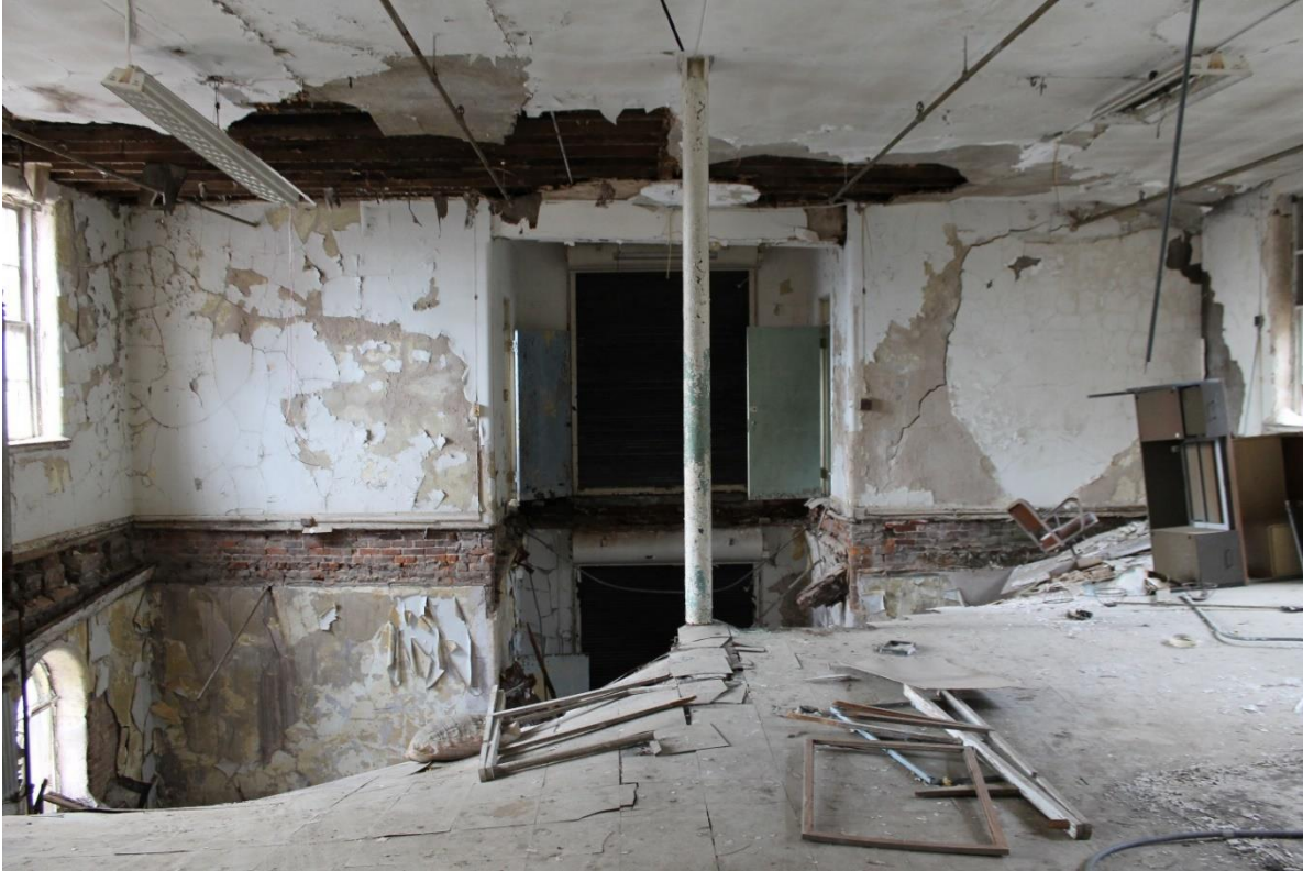
43. Northern wing, 2 nd floor, view to the south
