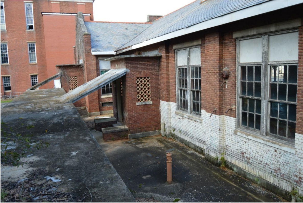
75. Men's dining hall, front, view to the northeast
