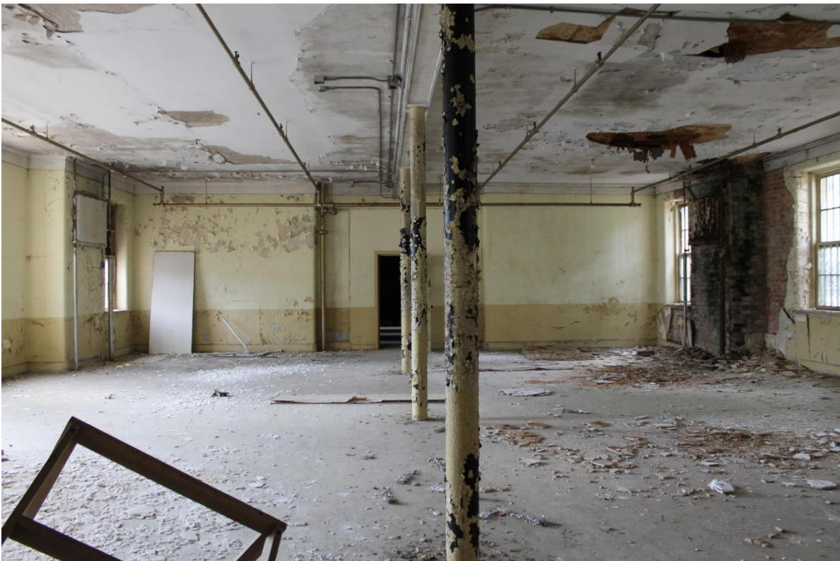
60. Southern north/south wing, upper level, view to the south
