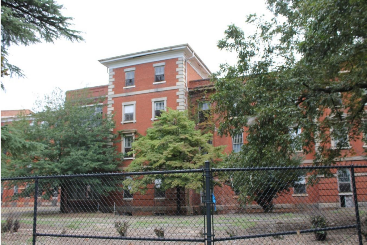
3. Northern north/south wing and first east/west block, view to the east
