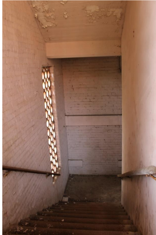
63. Sunroom addition stairs
