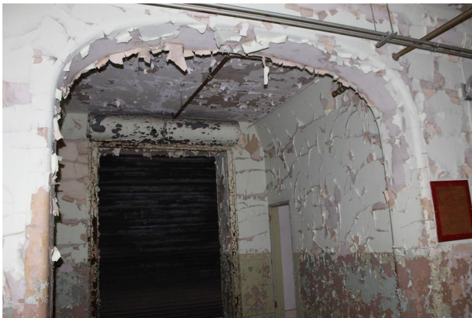
58. Southern east/west terminal block, opening to north/south wing, view to the north
