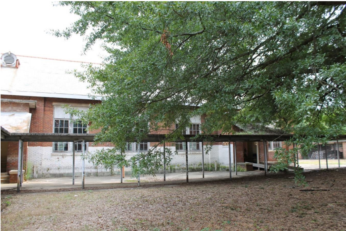
74. Men's dining hall, front, view to the east
