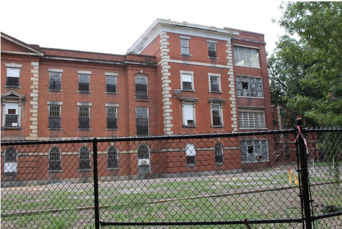
10. Middle southern east/west block and first north/south wing (on left), view to the southeast
