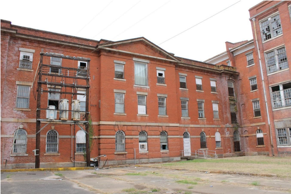
23. Rear (east side) of first north/south wing and middle east/west block, view to the northwest
