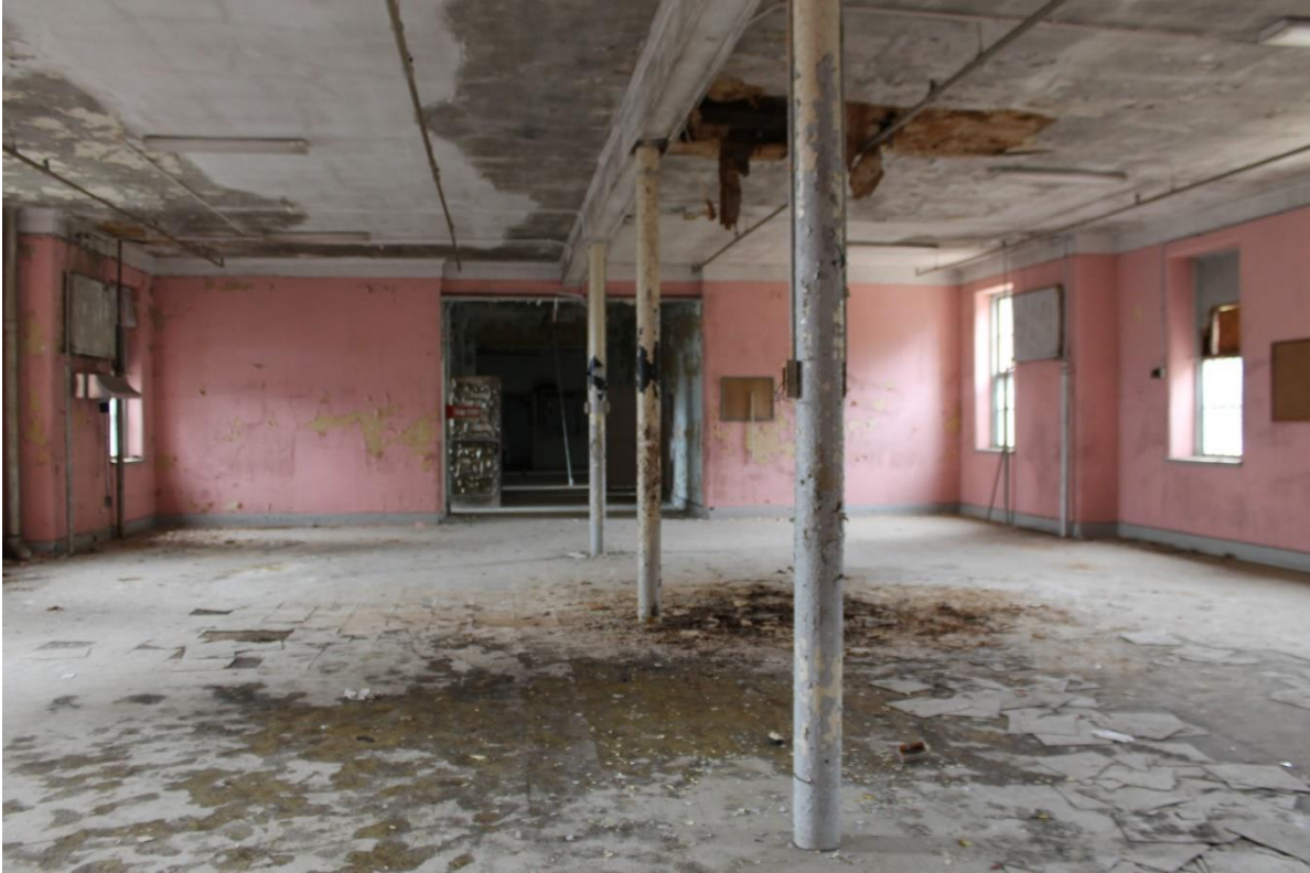
47. Northern wing, 1915 ward, view to the north
