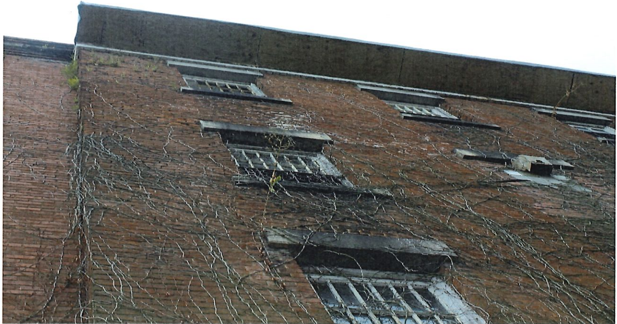
Photo 5 – Babcock Building 2150 Bull St. Columbia, SC New, temporary eave, southeastern corner of building 8/15/2019
