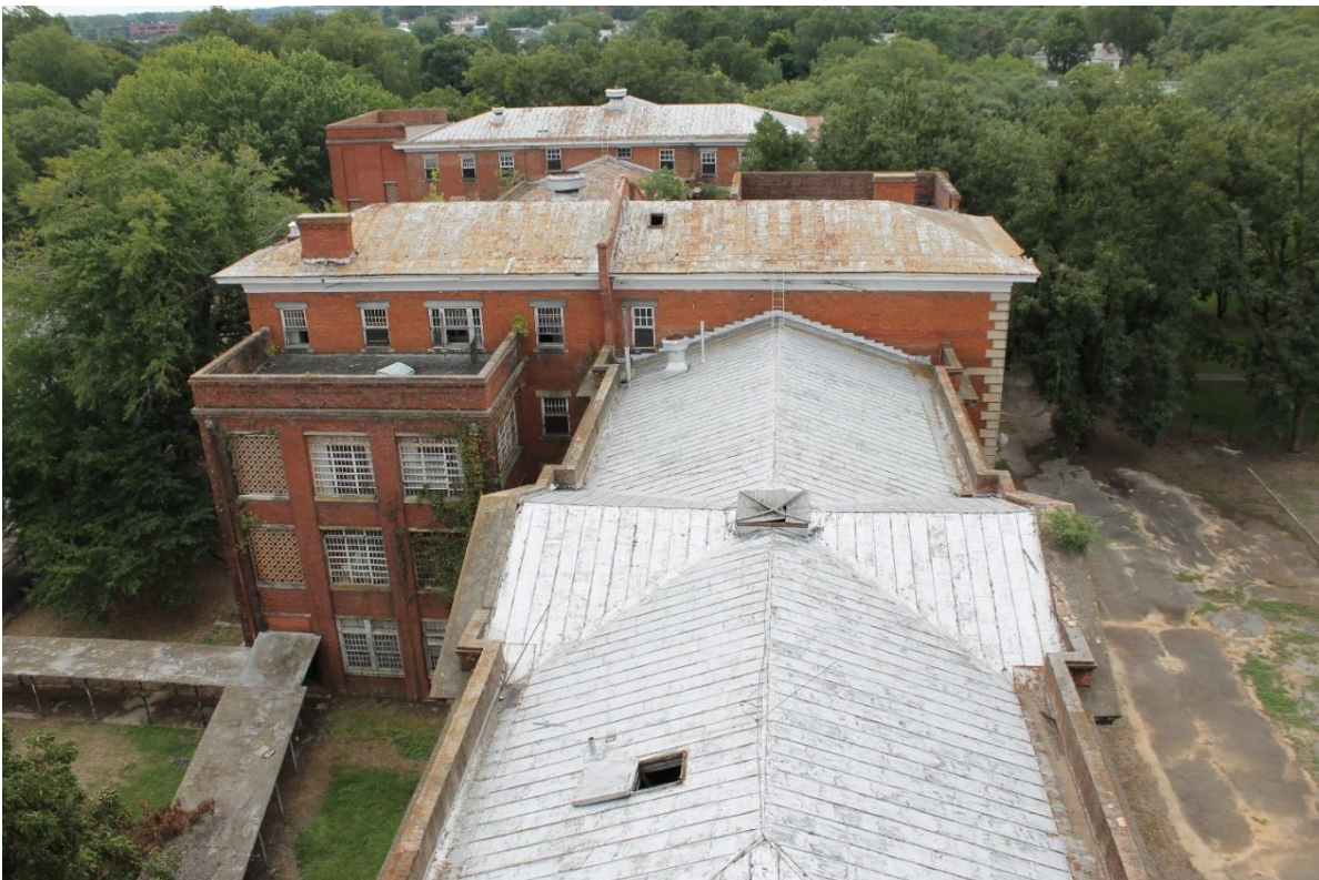
30. Roof of southern wings and east/west block, view to the south
