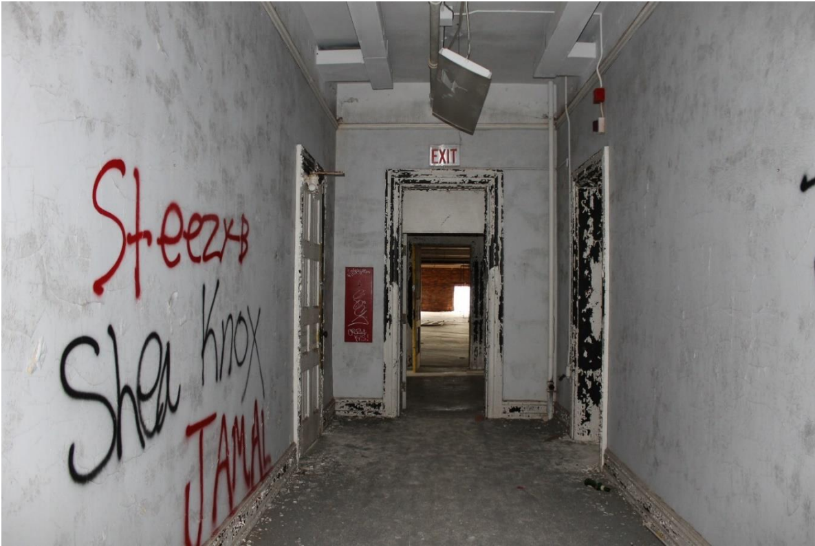
39. Center block, 4 th floor looking to the rear, view to the east
