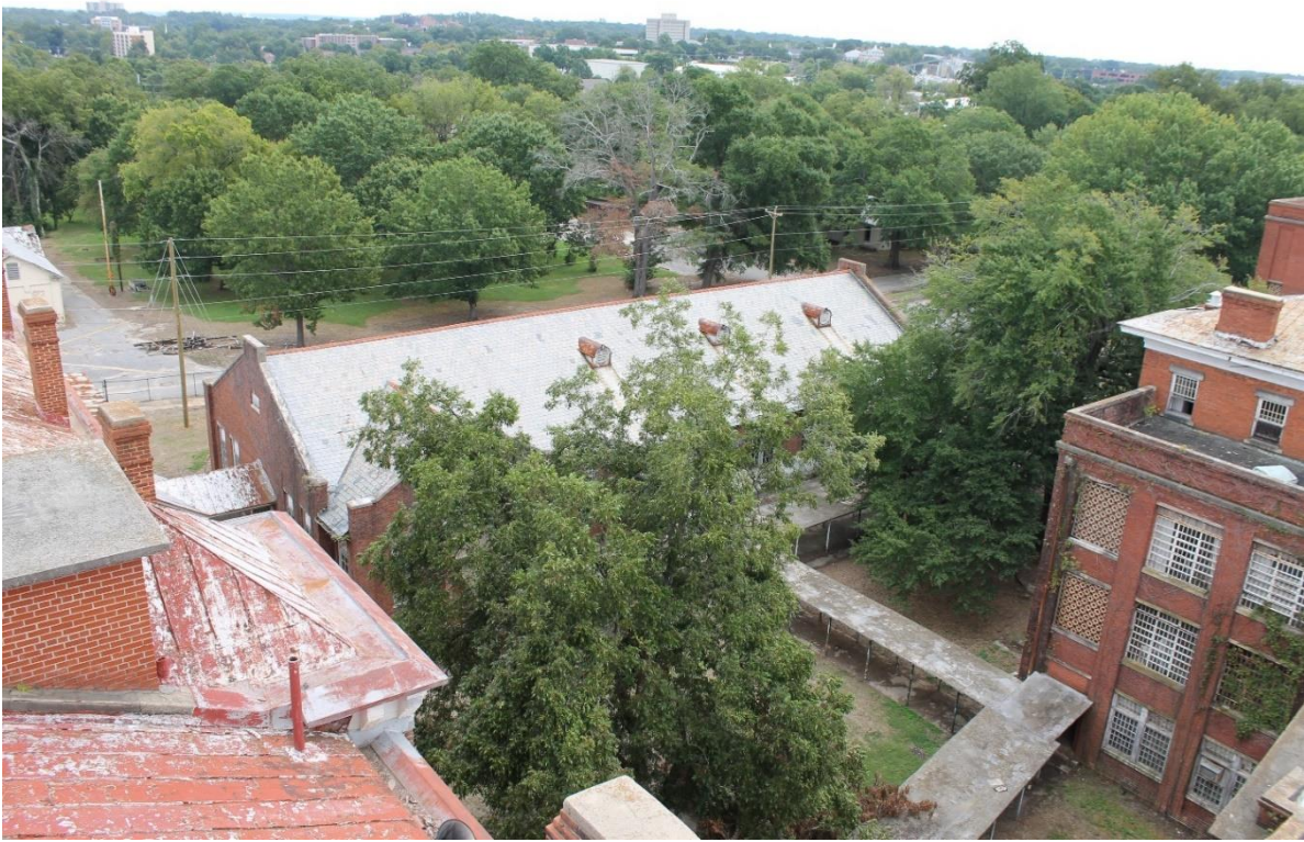
29. Men's dining hall and center section roofs, view to the southeast
