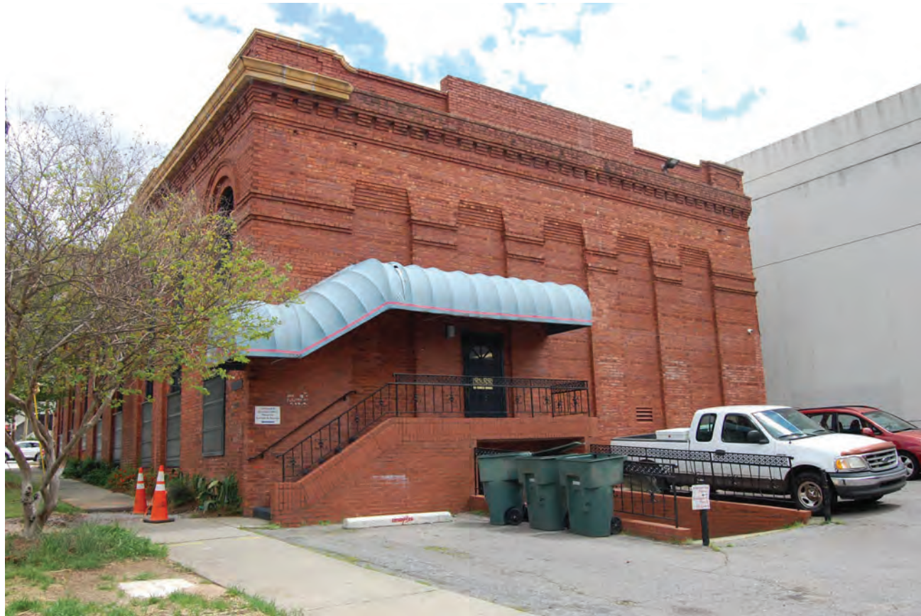
9. Existing West elevation of building.
