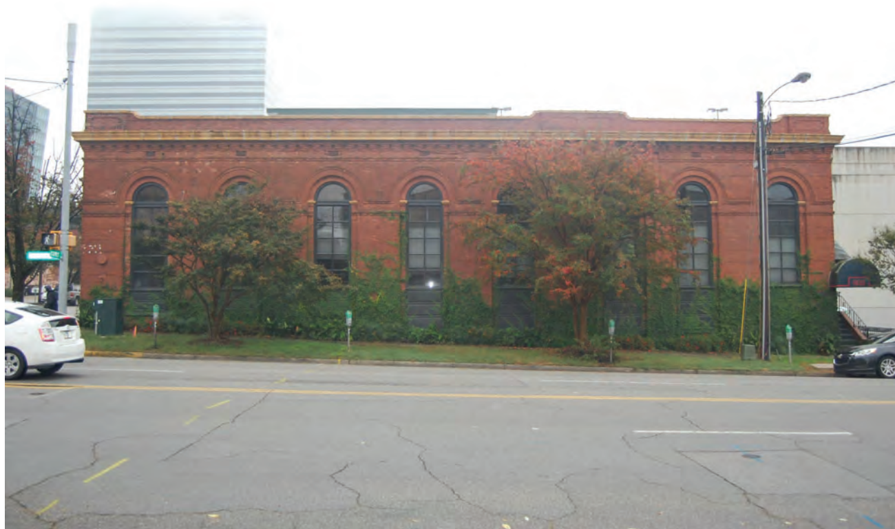
1. Existing North elevation of building.
