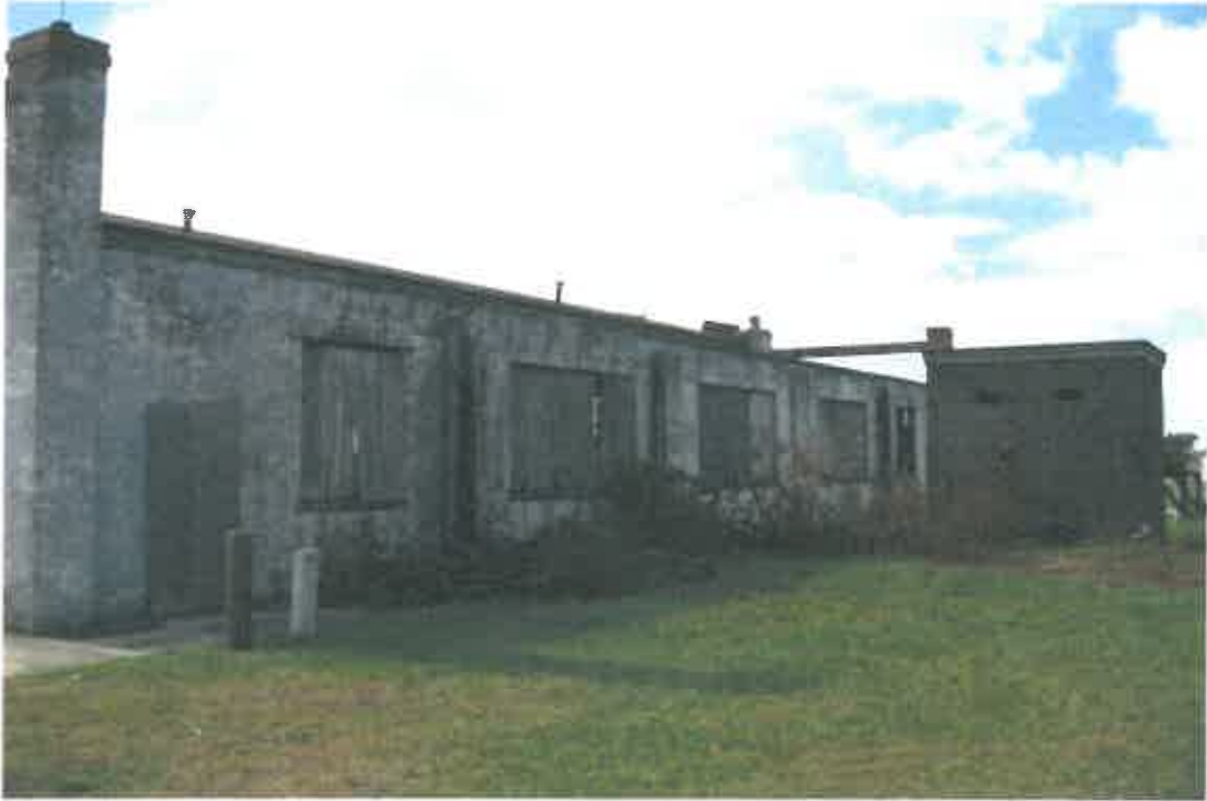
Photo 29 – Electrical outbuilding at west elevation
