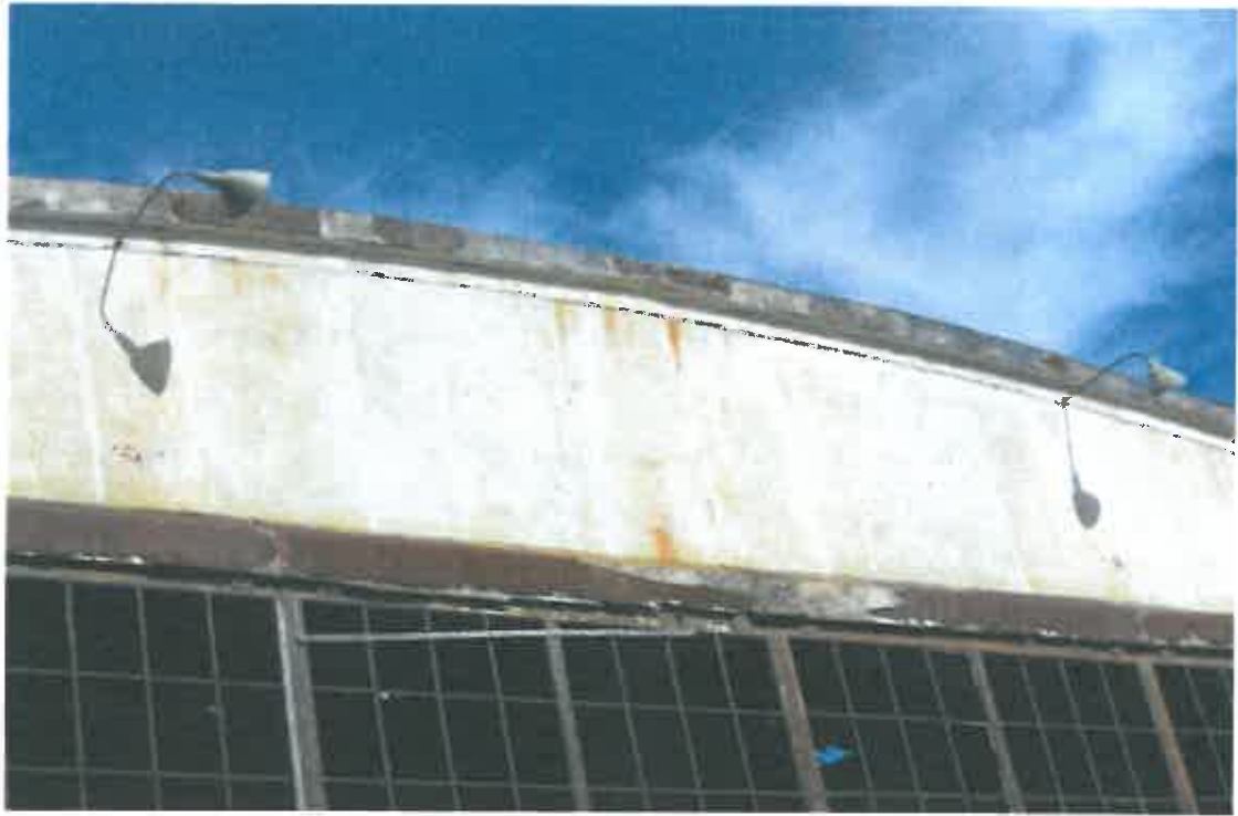
Photo 20 – Faded “Curtiss-Wright Flying Service” on south gable, with exterior light fixtures
