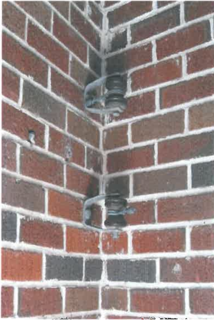
Photo 30 – Electrical outbuilding brick detail
