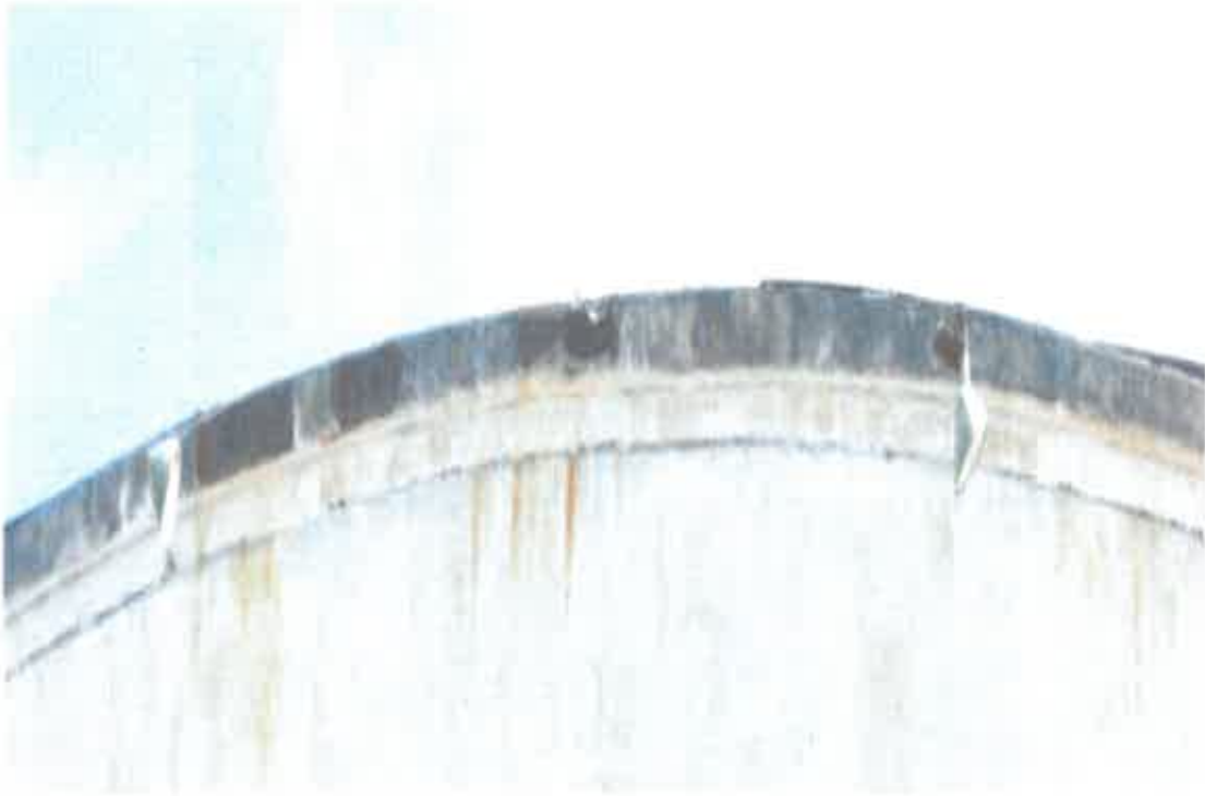
Photo 27 – Two exterior light fixtures, north gable
