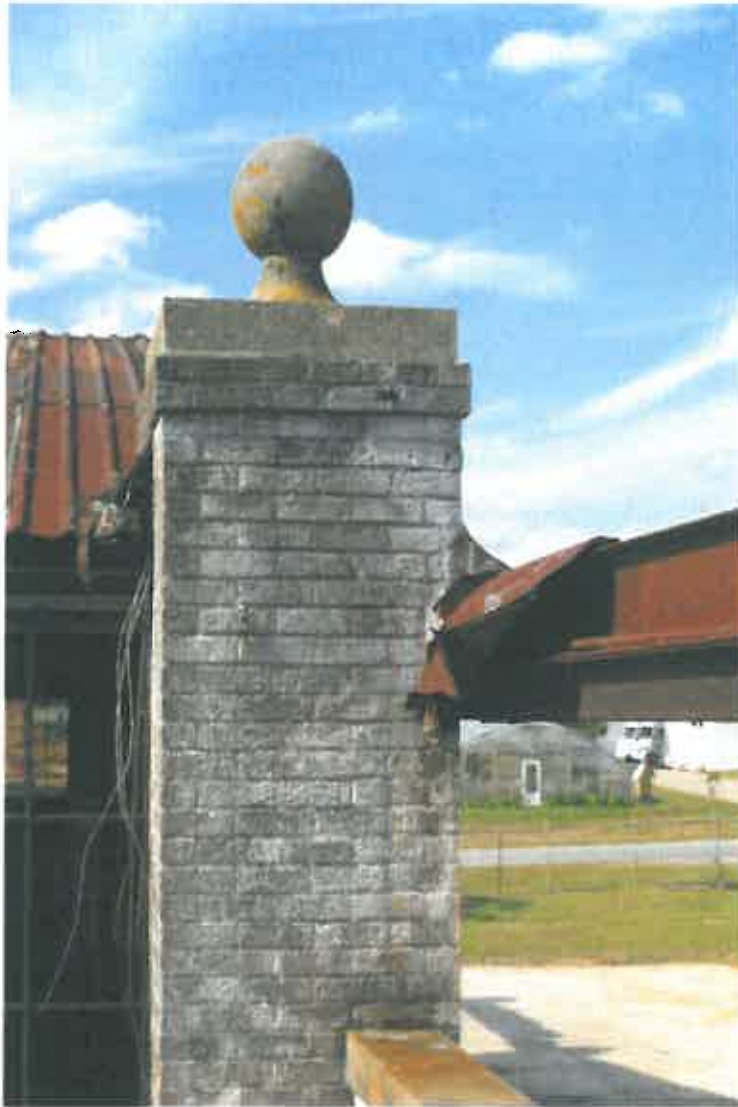
Photo 24 – Concrete finial, northeast corner
