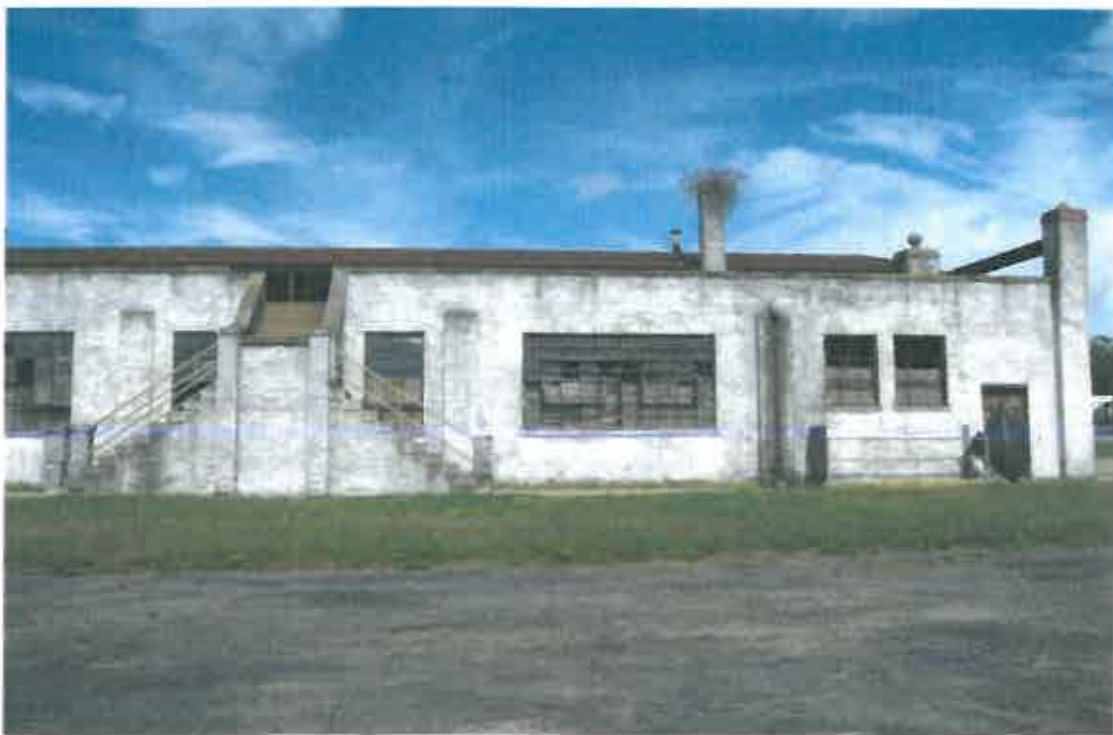
Photo 6 – View of roof, east elevation
