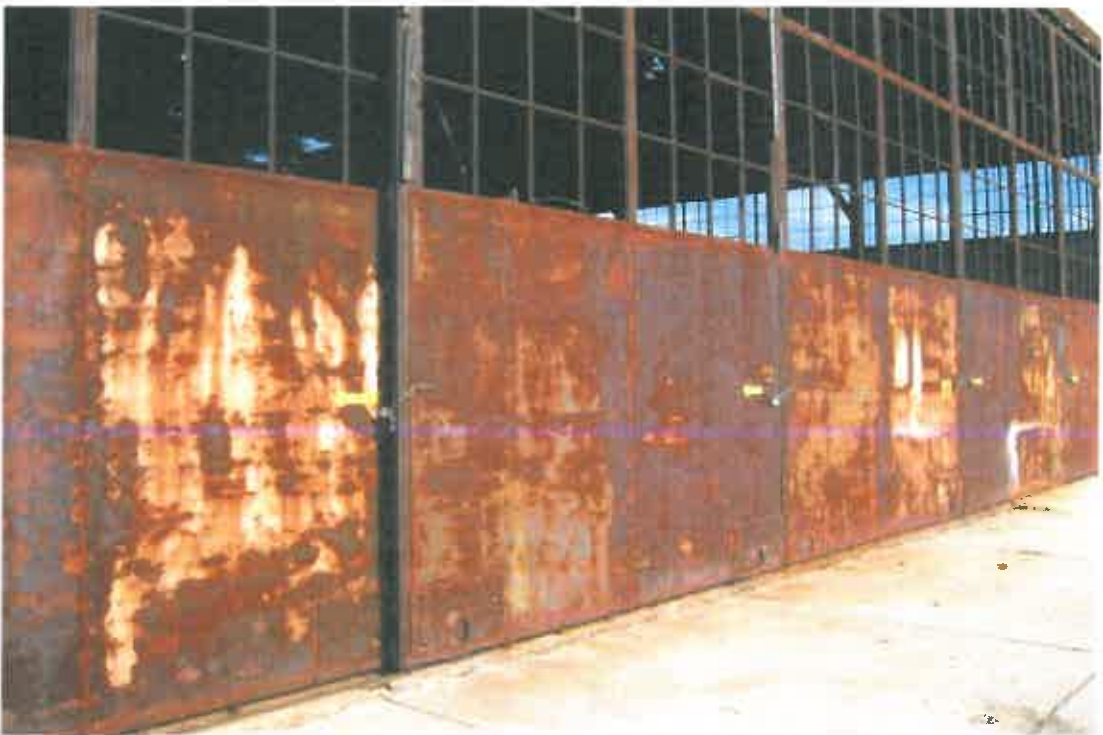
Photo 3 – Detail, hangar doors, south facade
