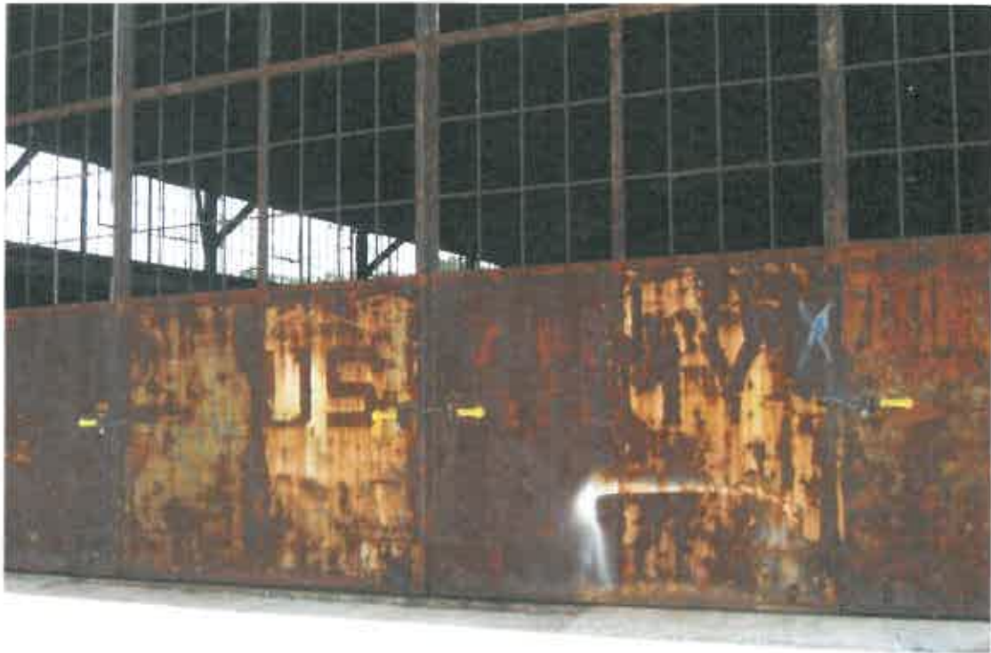
Photo 5 – "US ARMY" signage on south façade
