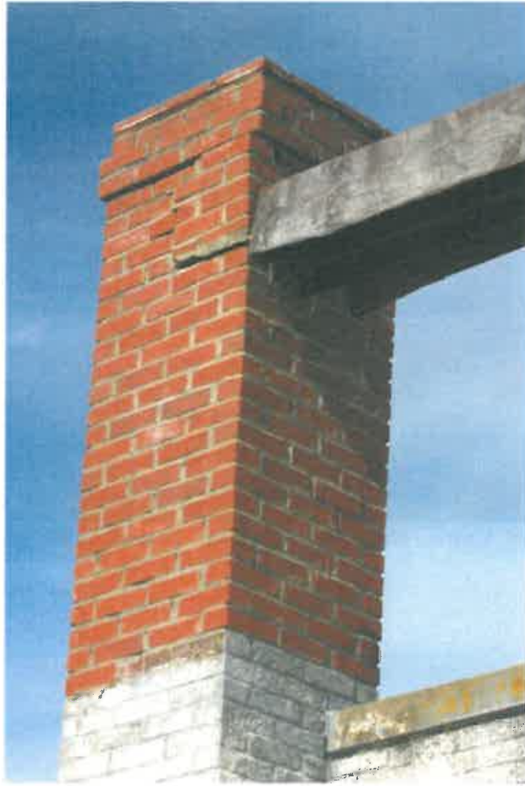
Photo 21 – Corner brick with truss
