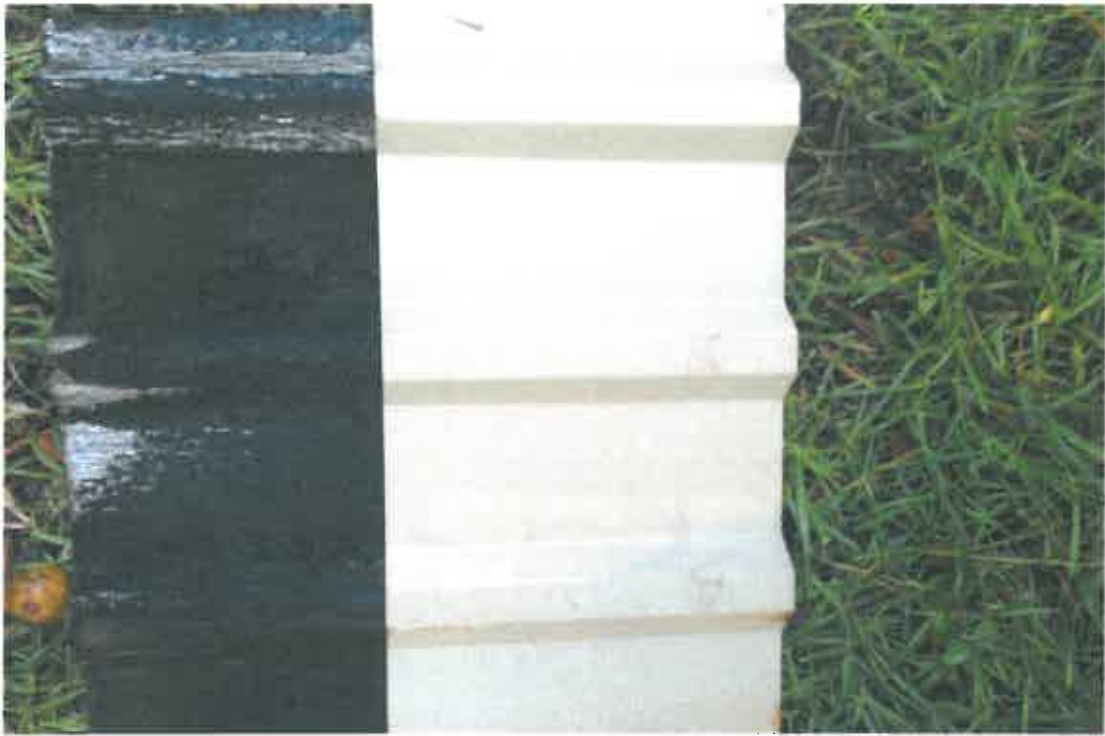
Photo 33 – New roofing panel compared with existing
