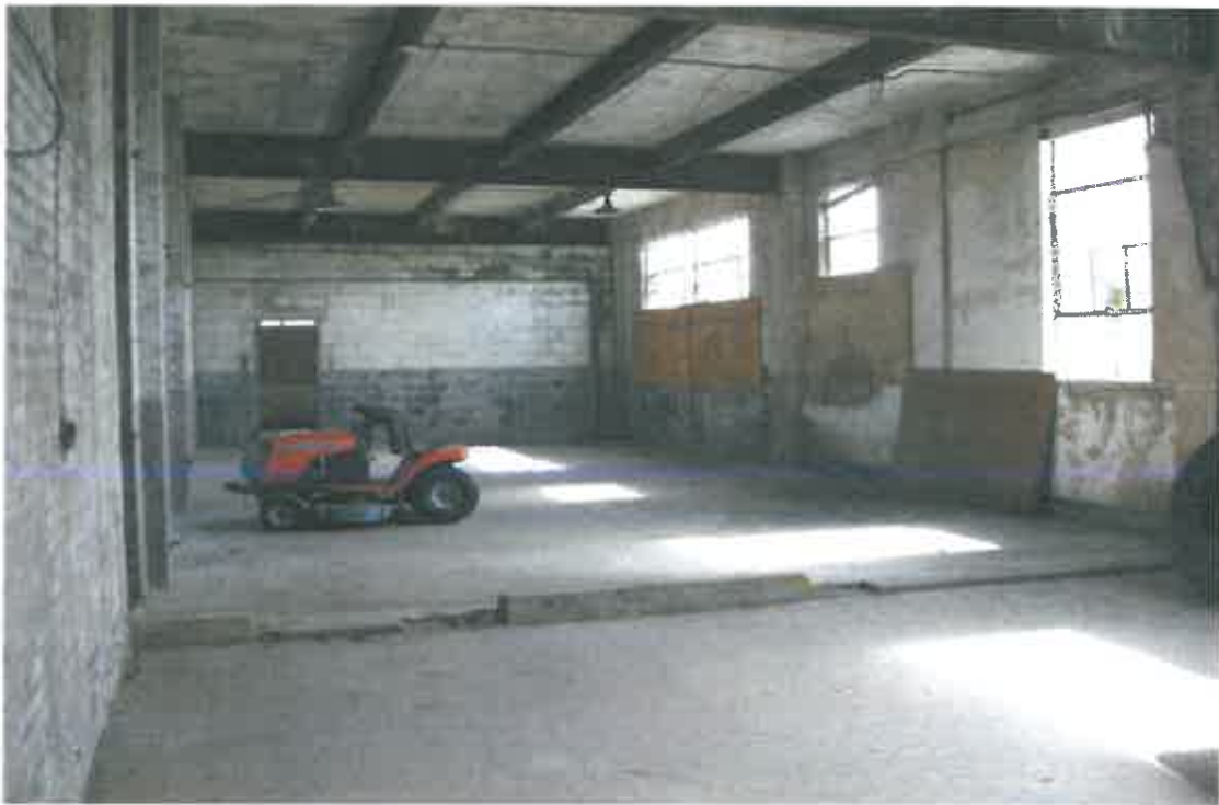
Photo 17 – Historic room divisions, east lean-to
