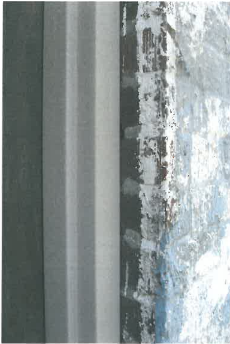
Photo 12 – Exterior brick detail
