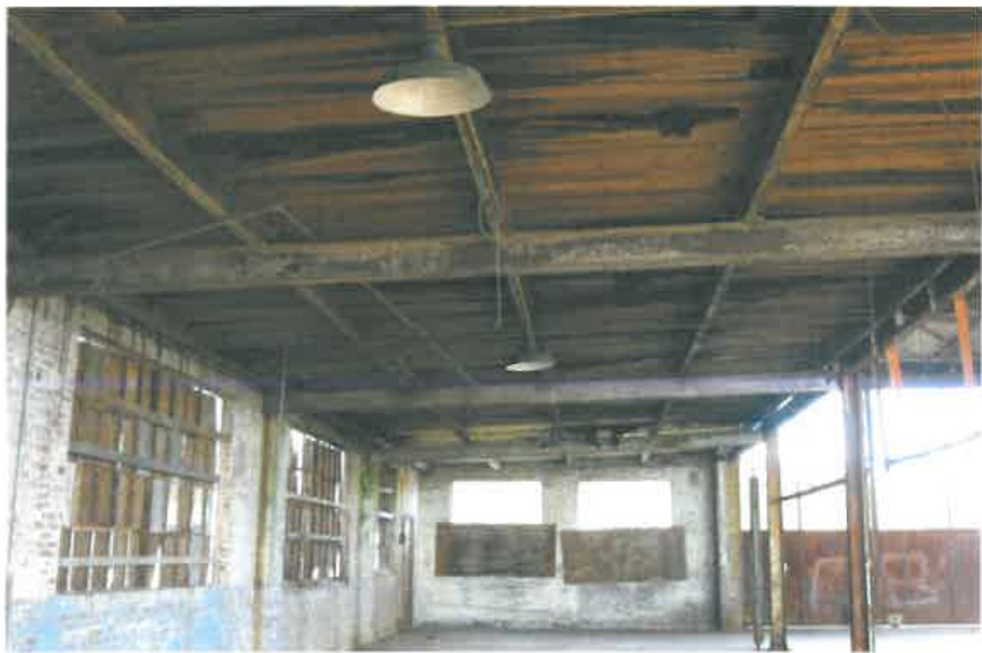
Photo 19 – West lean-to with interior light fixtures
