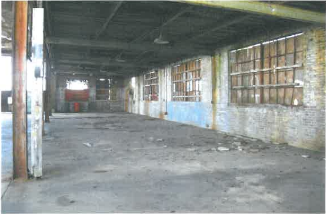
Photo 18 – Open west lean-to
