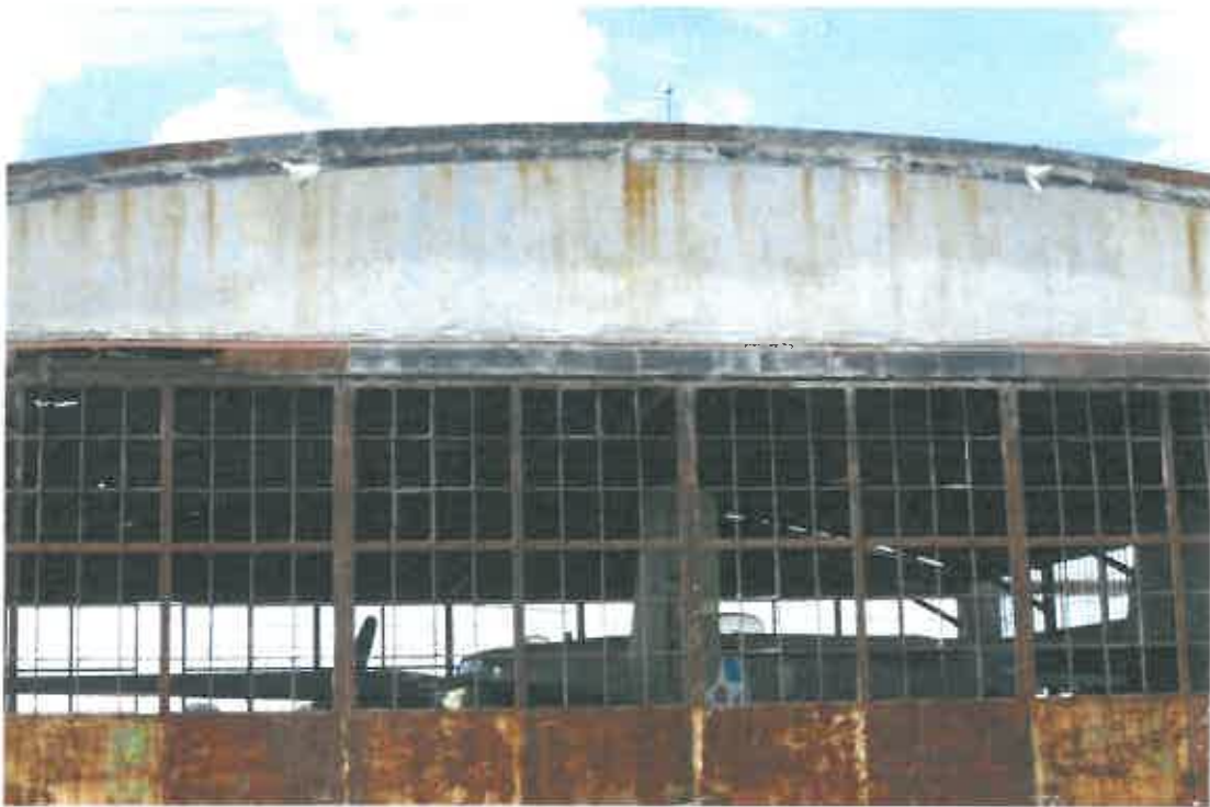
Photo 2 – Hangar doors, north elevation
