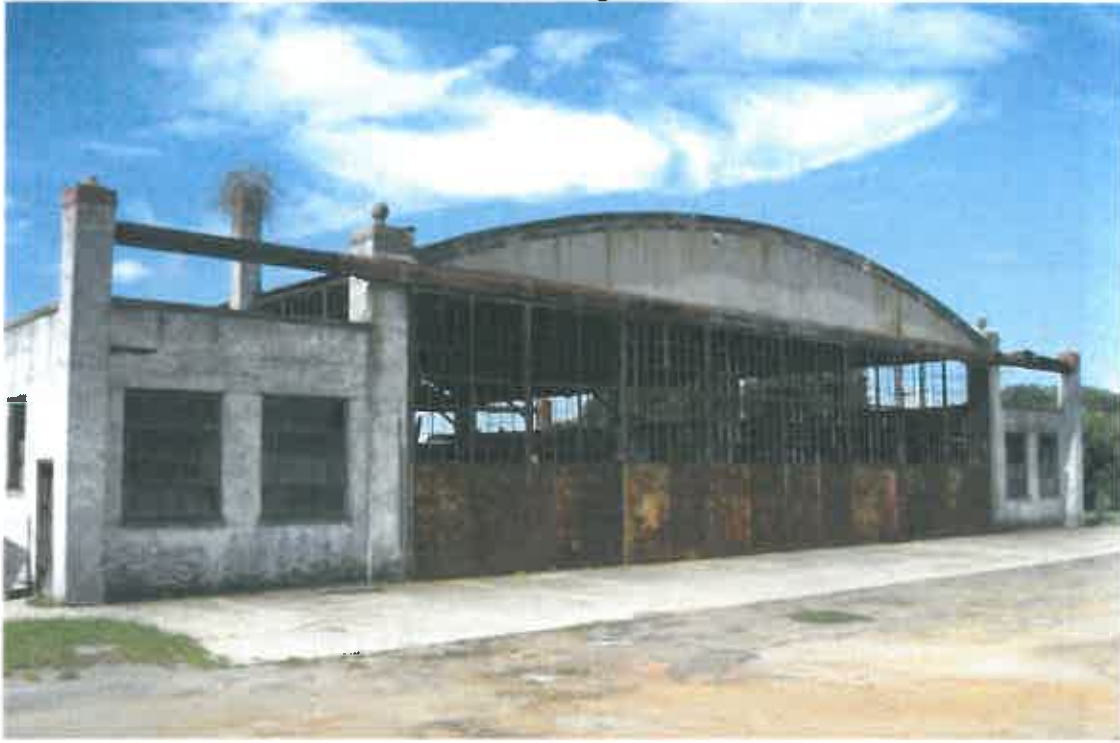
Photo 1 – Hangar doors, north elevation
