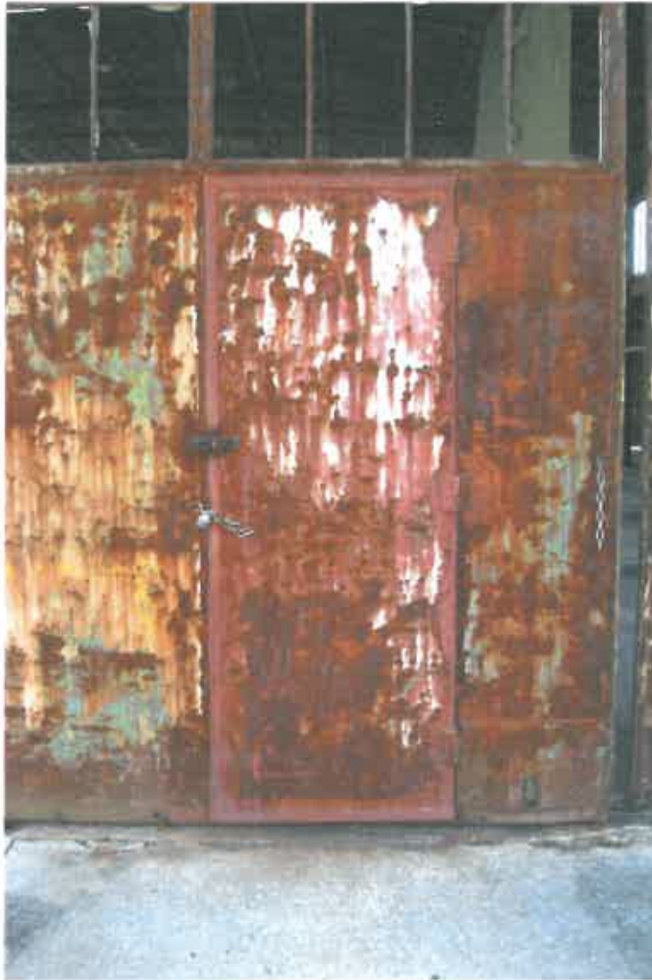
Photo 4 – Pedestrian door, north elevation
