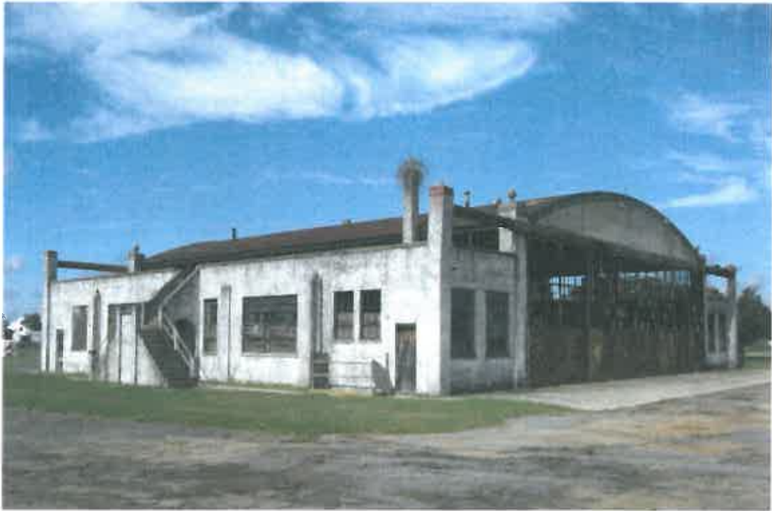
Photo 7 – View of roof, northeast oblique
