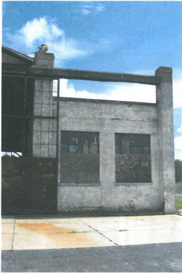
Photo 22 – Southeast corner columns
