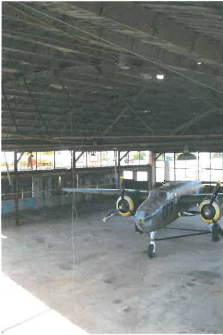
Photo 32 – Open space and exposed trusses
