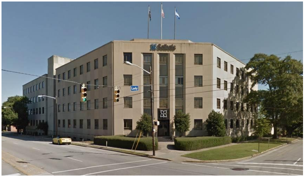
Google view of 1501 Lady Street, 1970s addition is seen at left
