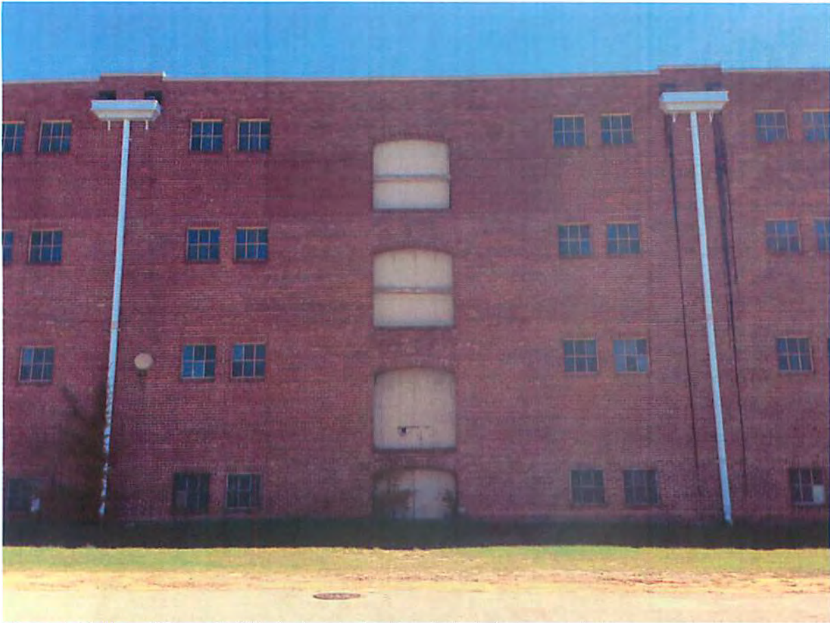
Photo 4: North end (newer building) of west elevation, typical windows and doors.
