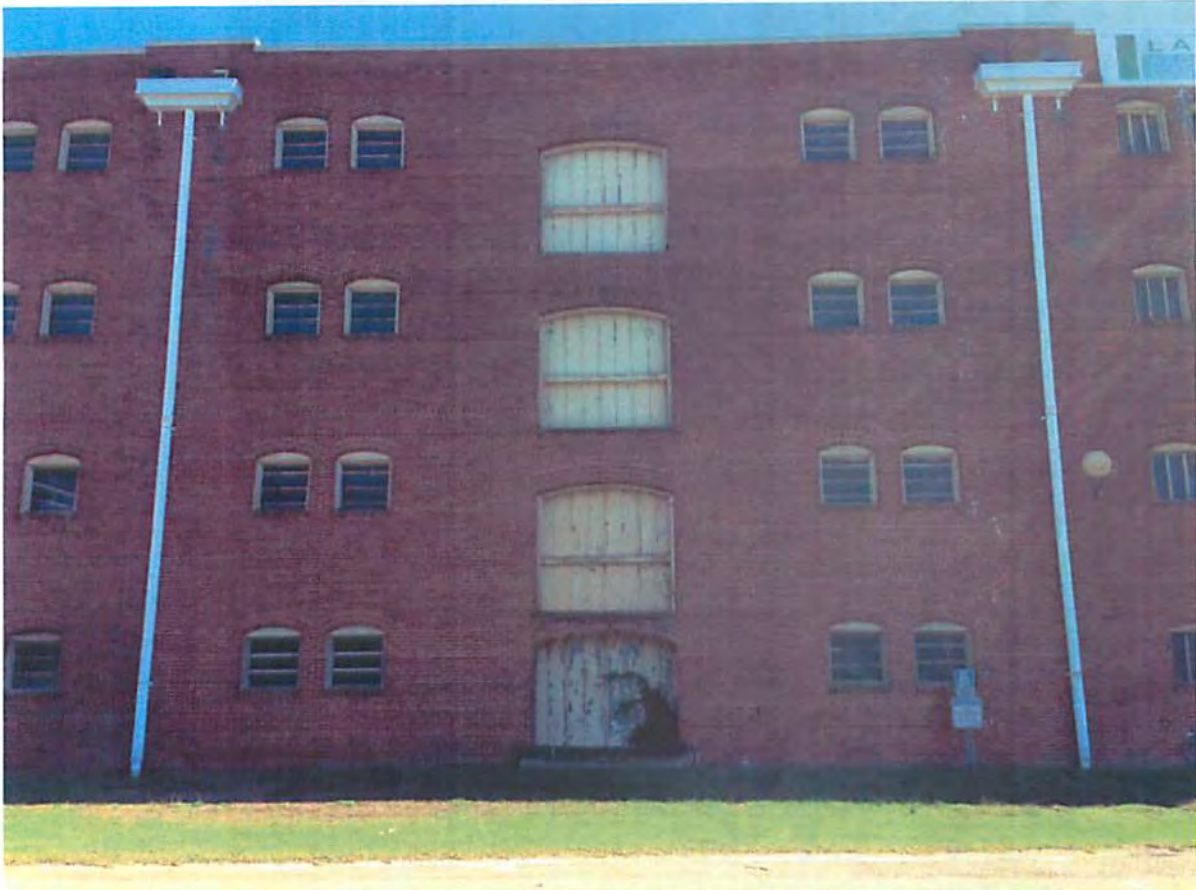
Photo 6: South end (older building) of West elevation, typical windows and doors.
