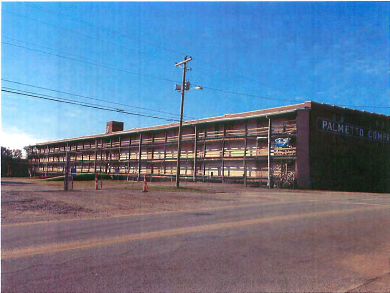
Photo 1: East elevation of PCW.
