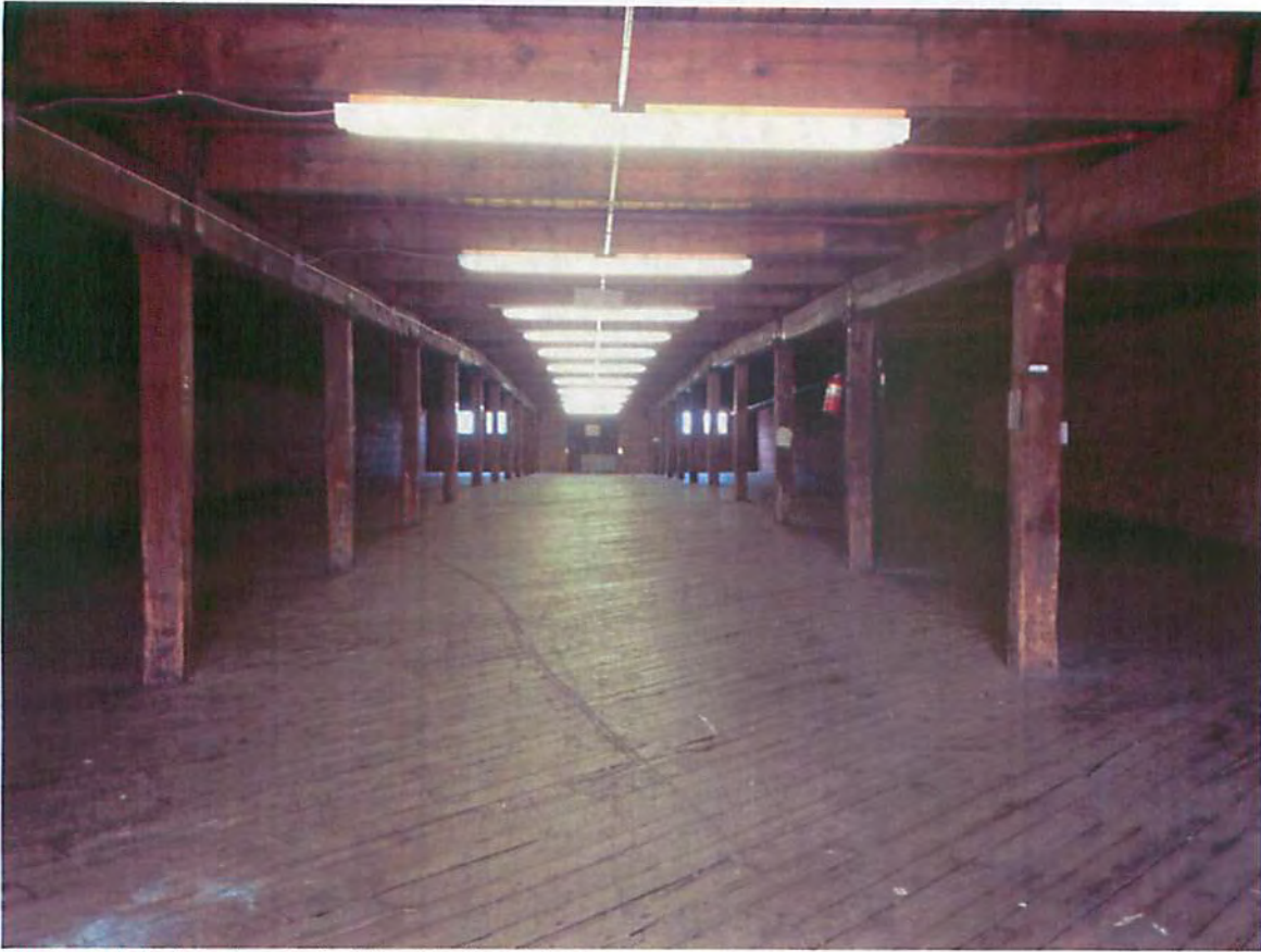
Photo 9: Interior view, typical bay looking West.
