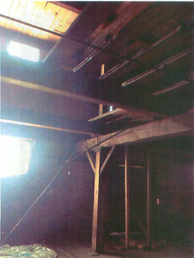
Photo 10: Interior view, previous demolition.
