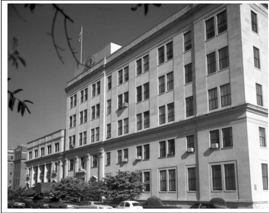
A 1979 image of the 1935 building by noted local photographer Russell Maxey. Image courtesy of Richland Library
