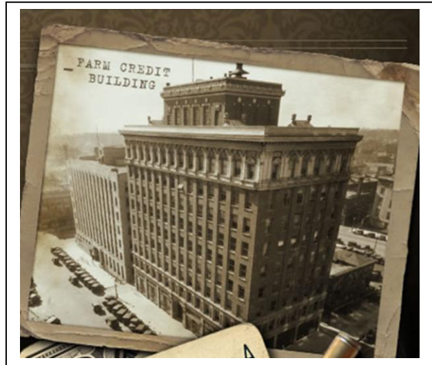
Built in 1923 and 1934 in Omaha, NE, this Federal Land Bank complex is now adaptively reused as apartments. Image from www.thebankomaha.com
