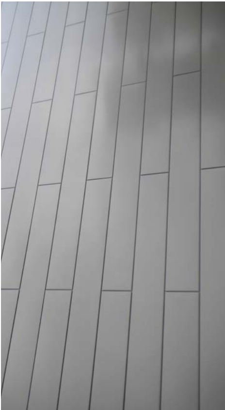
MTL-1 GARLAND ELEMENT MATERIAL HORIZ ARCH WALL PANEL SYSTEM W/ CONCEALED FASTENERS COLOR: PEWTER STAGGERED JOINTS
